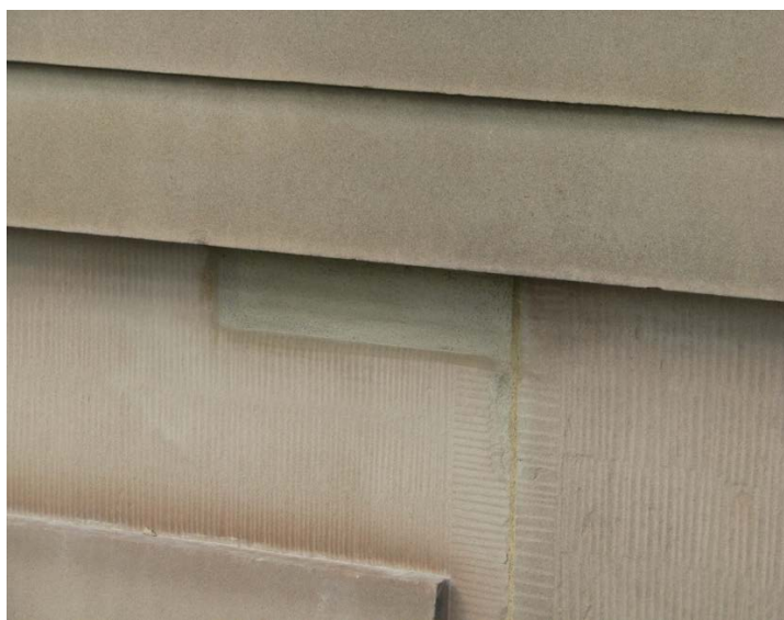
View of sandstone fine jointing work and repairs, Province House NHS
