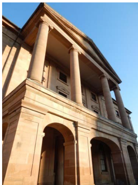
Angled view showing Ionic columns, above and Doric piers with decorative pilasters, below.
