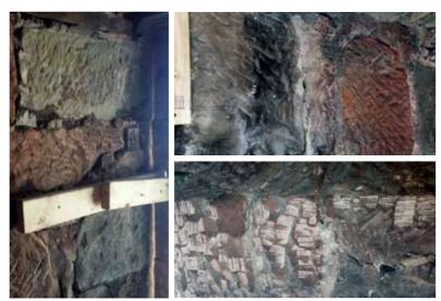
In these photos, you can see the individual chisel marks on the stones used in the original construction of the building. Each stone was shaped by hand, using a variety of different chisels and, as you can see, each mason had their own preferred technique.
