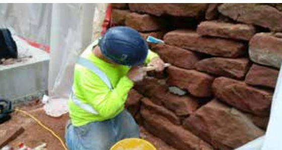
Foundation Island stone after deep raking (left) out and deep joint and void filling in progress (right). Photos courtesy of HCS, 2017
