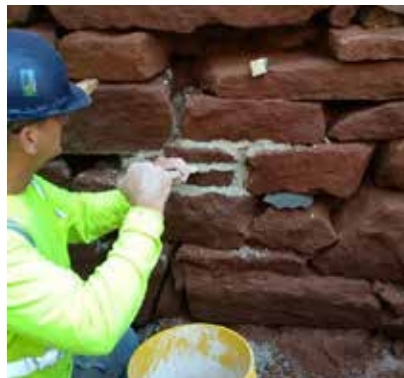
Completed in situ repair test.
