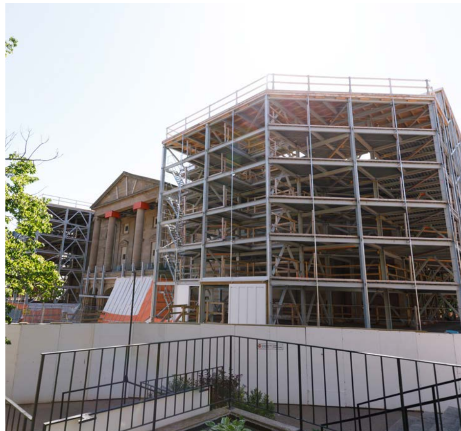
View from west of Province House, 2018 ©Parks Canada
