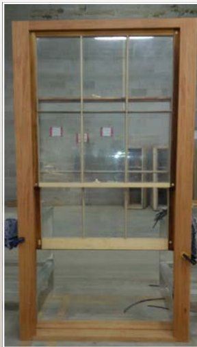
Repaired window frame and sash (April 2019)
