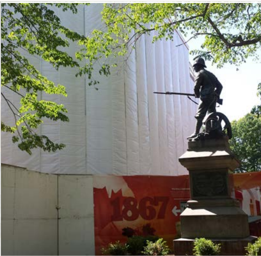
East exoskeleton fully clad with sailcloth (June 2019)
