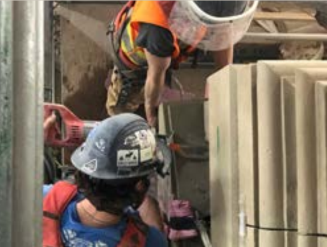
Two masons working within tight quarters as they install an exterior stone.
