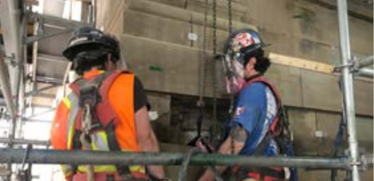
Two masons wearing full Personal Protective Equipment (PPE) along with face shields as they install a stone.
