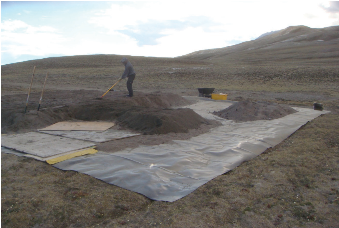
Photograph IV-8: Construction of the Lake Hazen landfarm: addition of the 30 cm layer of hydrocarbon-contaminated soil.
