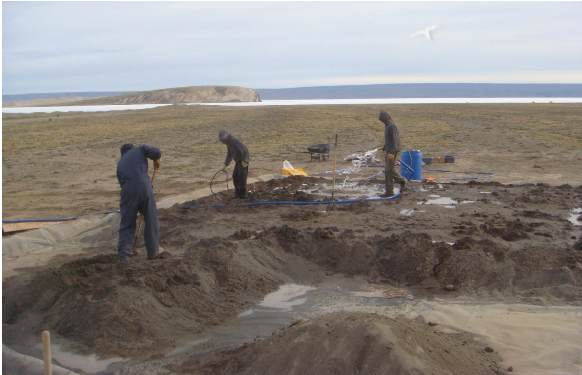
Photograph IV-11: Landfarm treatment: fertilizer and Biosolve ™ were mixed into the soil, which was homogenized using a shovel.
