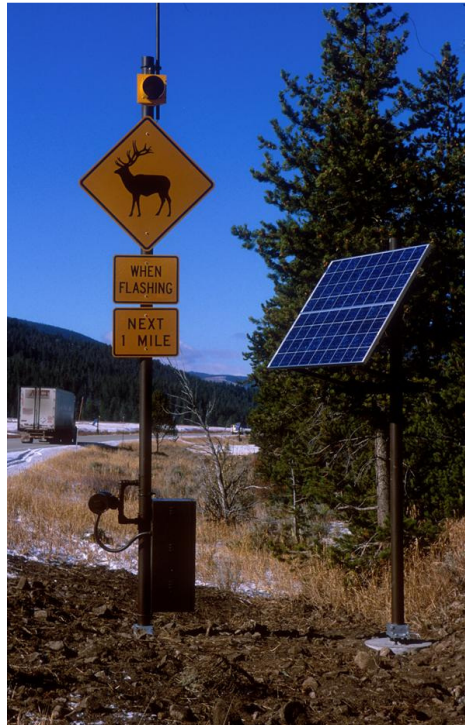
Animal detection system along Highway 191 in Yellowstone National Park, Montana (Photo: Marcel Huijser, WTI).
