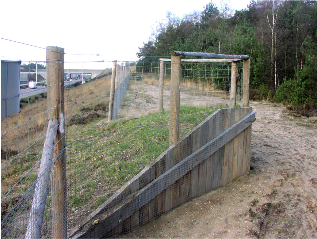
Wildlife "jump-out" escape ramp (Photo: Tony Clevenger).
