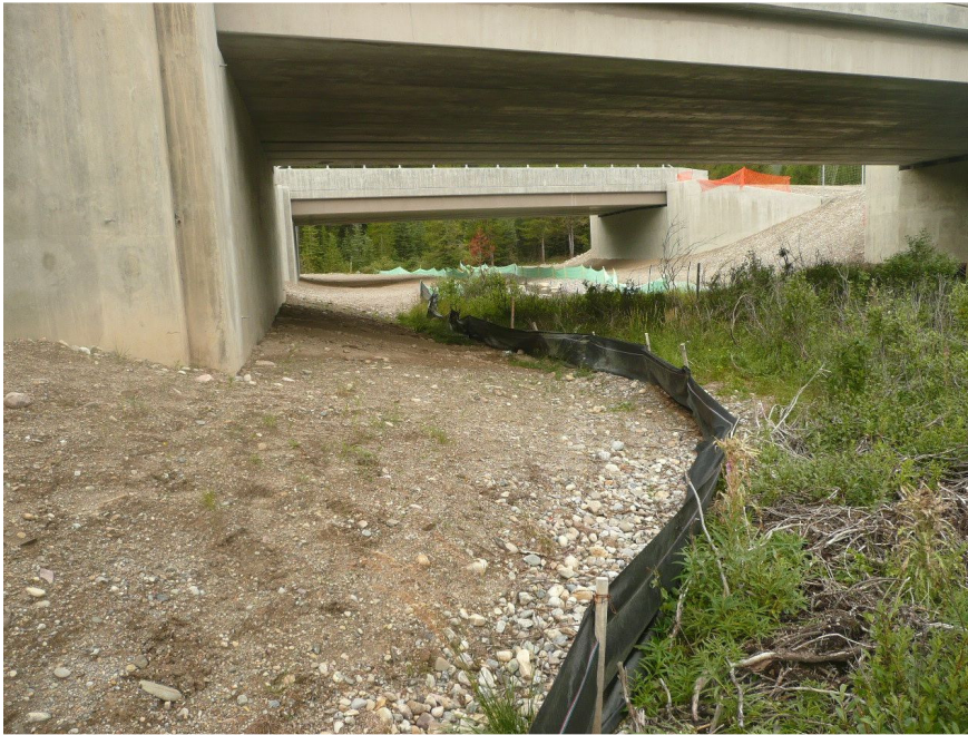
Figure 7.2: Example of 22 m wide wildlife underpass, Trans-Canada Highway, Banff National Park, Alberta (photo credit: T Clevenger).
