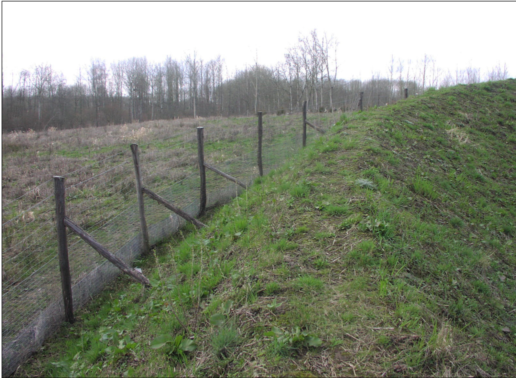
Berm on wildlife overpass (Photo: Tony Clevenger).
