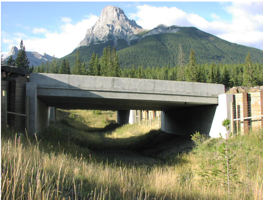
Figure 7.1: Open span wildlife underpass on Trans-Canada Highway near Dead Man’s Flats, Alberta (photo credit: T Clevenger).
