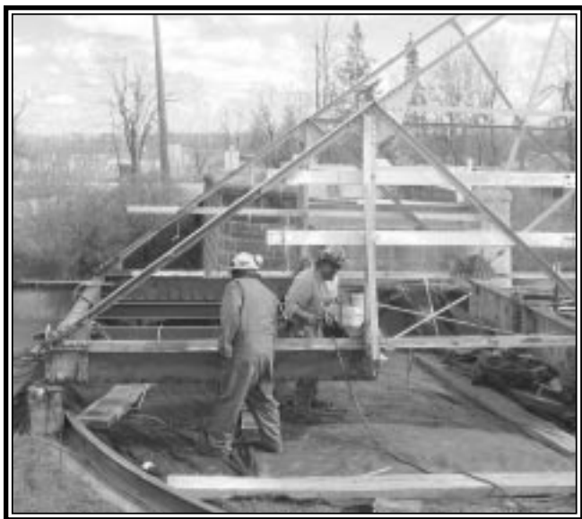
Burritt's Rapids Swing Bridge Bill Pratt
