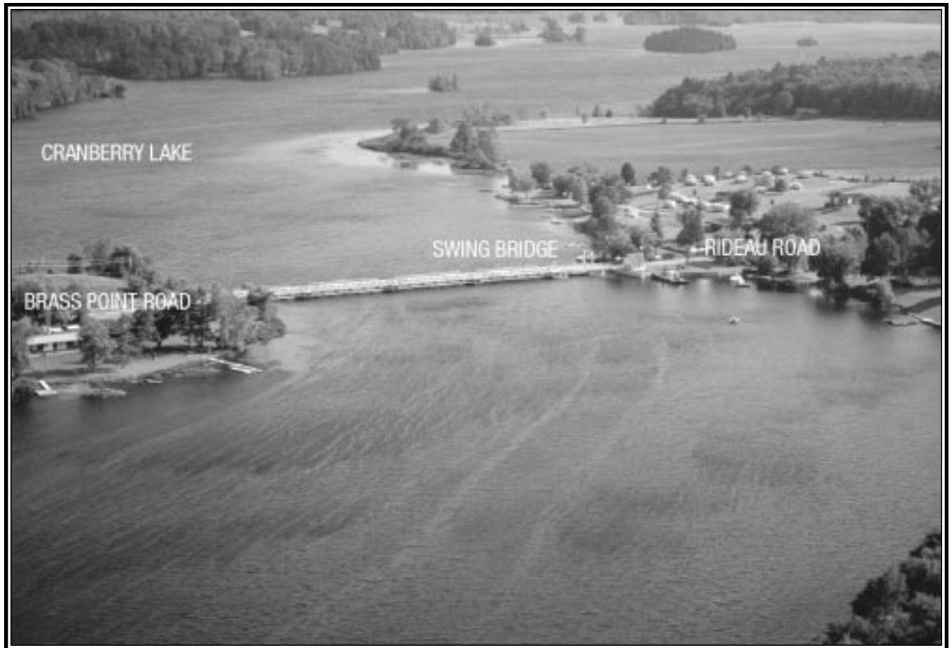
BRASS POINT BRIDGE
