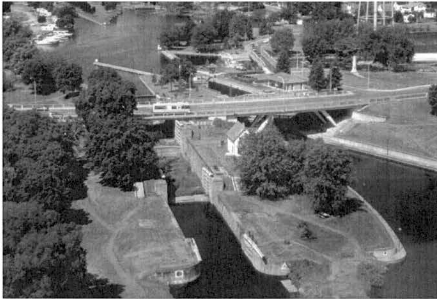
Figure 1: on left hand side, original lock and on the right is the new lock 29A
