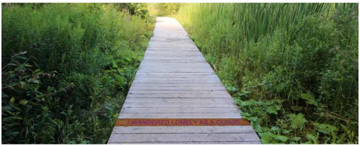
Poetry integrated into wood boardwalks using water-jet cut Corten steel strips with an optional purple backing
