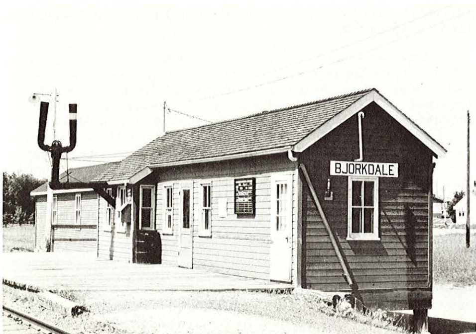
The Bjorkdale depot, located on the line from Reserve to Crooked River, is one of the few portable depots left in Saskatchewan. While the CN built this particular station, it is typical of portable depots in general. In this small, narrow structure are the three distinct sections of the standardized depot: waiting room, center agent's office, and freight-baggage-express area.
