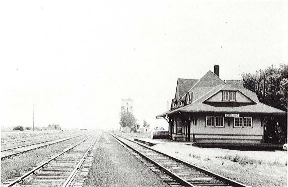
The Kipling depot, southeast of Regina on the line from Regina to Winnipeg, is an example of an early Second-Class station design. The hip dormers on the ends and sides make this building much less massive in appearance than the later Radville depot. Kipling is a division point that still has a small yard; it once had a roundhouse.
