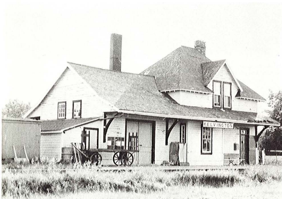
Kelvington is located in east-central Saskatchewan. This building is typical of the CNoR Third-Class depots. The high-hip roof, the gable dormers, and the bracket-supported shingle awning are all easily recognized. The bay window is nearly hidden by the awning. The small lean-to-like addition on the end was used as a coal bin; some stations lack this feature.
