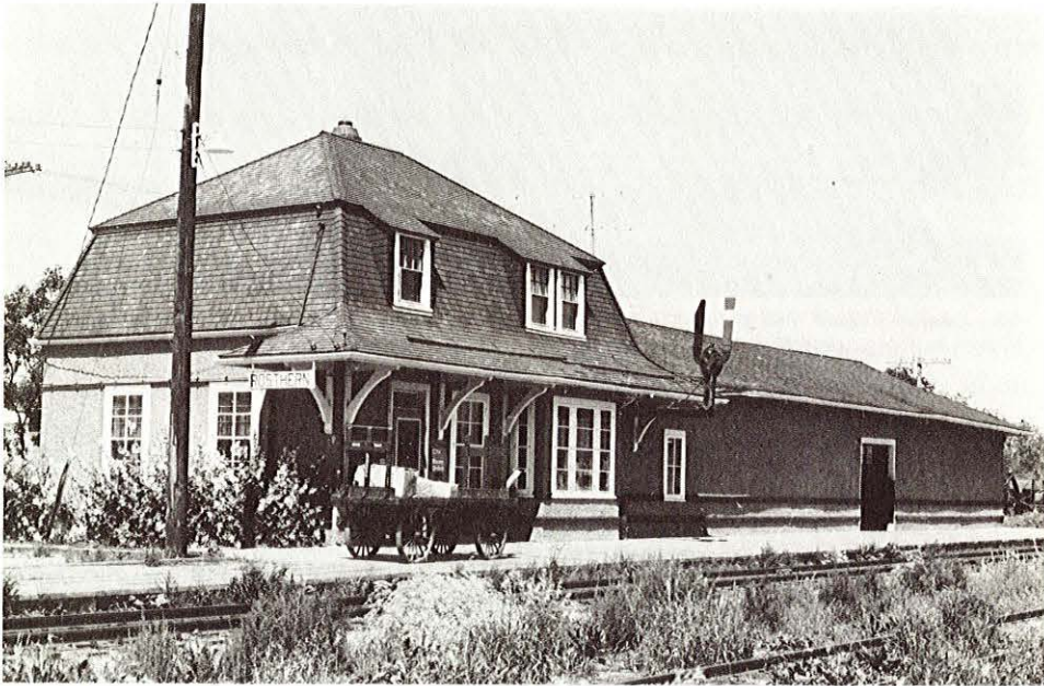
The Rosthern depot, built in 1902, is north of Saskatoon on the QLL&S. It has the distinctive hip-gambrel roof which sets it apart from other CN depots in Saskatchewan. The white brackets supporting the shingled awning can be readily seen between the bay window and waiting room.
