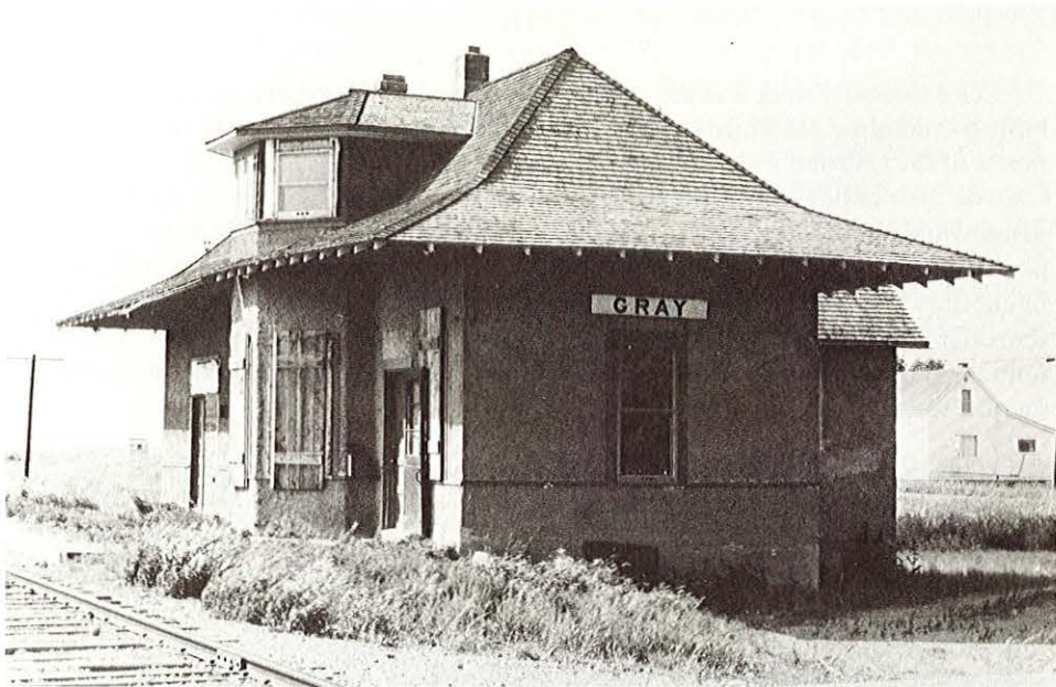
The Gray station is southeast of Regina on the line to Northgate. The small addition attached on the rear of the depot, visible in this photograph, is the kitchen. By confining the agent's living quarters as much as possible to the rear section and second floor, depot additions could be made without having to relocate the living quarters.
