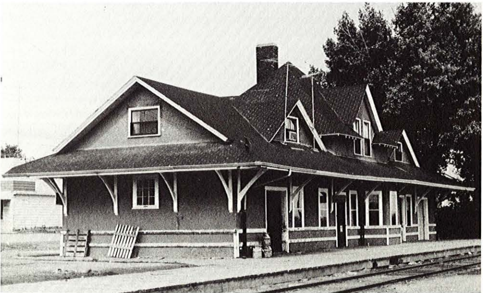
The Radville station is southeast of Weyburn. This depot was constructed in 1912 and is typical of Second-Class stations located on lines built after 1910. While later depots retain the pyramid roof on the center section, awning, and bay-window design of earlier ones, the gable dormers on the ends and sides make the Kipling and Radville buildings appear different. The wood strips that run parallel to the ground on the lower portion of the station are designed to protect the stucco from chipping by baggage wagons and other vehicles. Radville is the junction for several lines and once had a roundhouse. Another station similar to Radville's may have been located at Kindersley.
