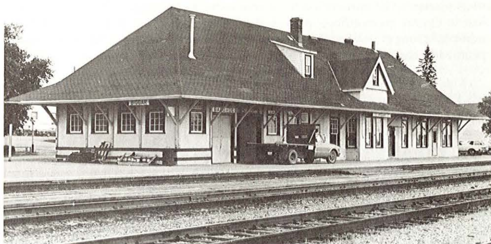
Biggar is a division point on the CN mainline west of Saskatoon. To accommodate the needs of a division point, a larger standard depot was built. The station at Watrous, also a division point, is a similar structure.
