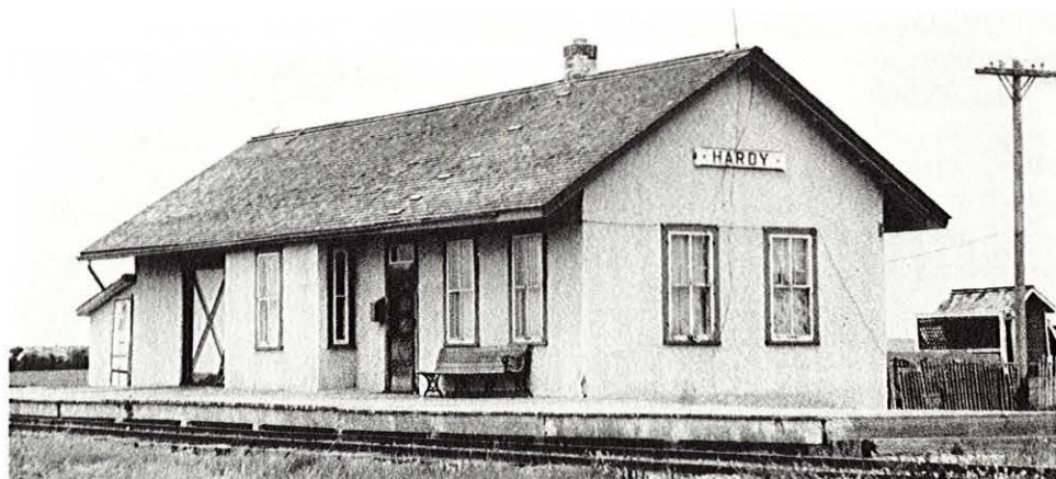
The Hardy station, built in 1920 and located in southwestern Saskatchewan near Willowbunch, is a marvelous example of the CNoR Fourth-Class depot. The wooden platform, used almost exclusively in Saskatchewan, is evident in this photograph.
