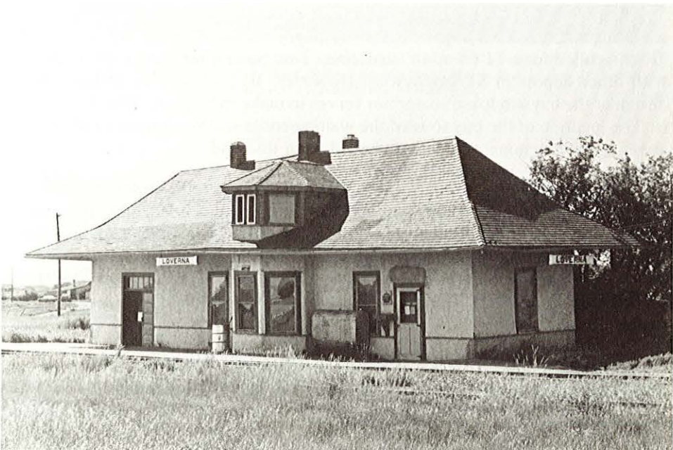
Situated in west-central Saskatchewan on the line from Biggar, the Loverna depot is another example of how a standard depot could be altered to meet local needs. For an unknown reason the company decided that Loverna needed a longer waiting room. The standard plan the GTP used for stations like Gray easily accommodated this need.
