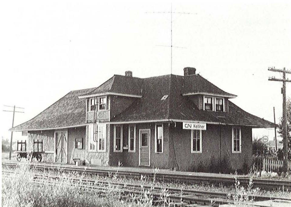
Kelliher is located in south-central Saskatchewan on the CN mainline. This station is wider than the other GTP depots already discussed; it contains an extra window on the waiting-room end. The flat deck over the office and waiting room is so well hidden that one must look closely to find it; the TV antenna is mounted on the deck. This deck extends from just behind the end dormer to the freight house.
