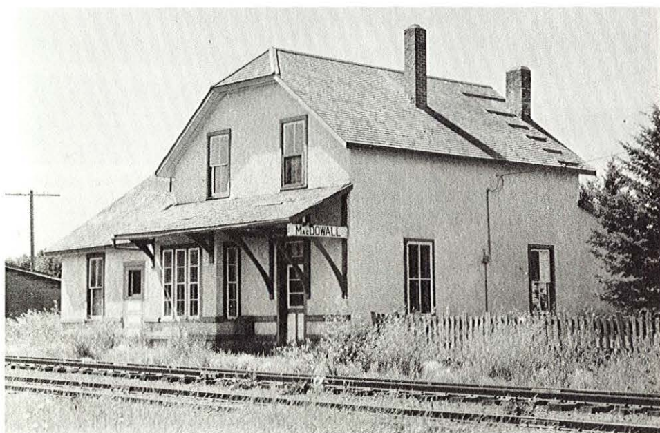
MacDowall is north of Saskatoon on the QLL&S. This station built in 1891 appears to be a smaller version of the Dundurn depot. The hipped-gable roof over the second storey, the gable roof over the freight house, and the shingled awning along the front of the waiting room and office are features found on the larger Dundurn station. Railroads in Western Canada did not hesitate to borrow from one depot design to apply to another. Only five depots like the MacDowall structure were found in Saskatchewan in the 1970s, all along the QLL&S.
