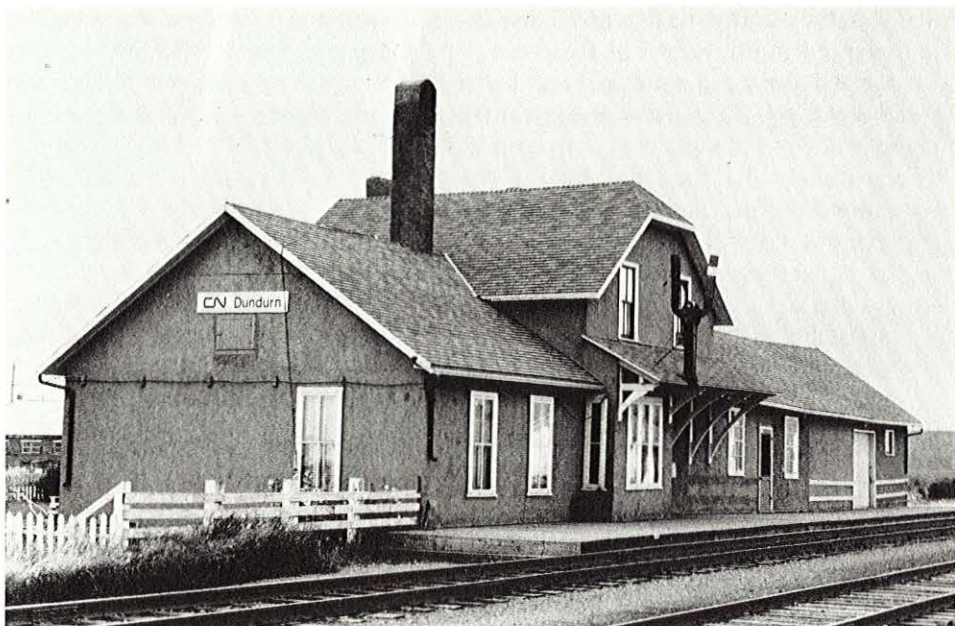
The Dundurn depot, constructed in 1892 by the QLL&S, is a fine example of one of the earlier CN depots built in Saskatchewan. The only other depot like it in the province is located at Craik on the same line.
