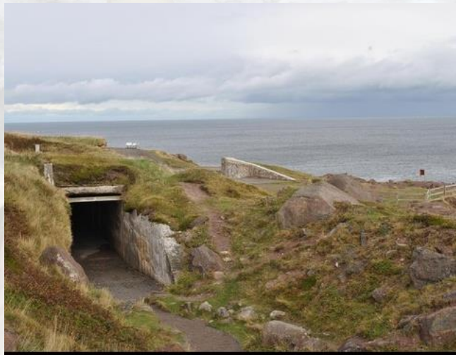
Figure 6. Cape Spear WWII bunker.
