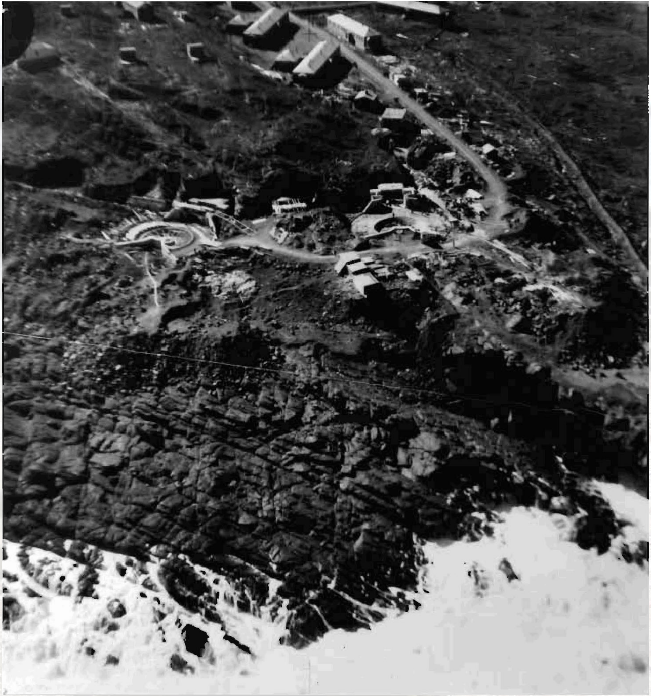
Figure 15. Aerial view of gun battery at Fort Cape Spear under construction in 1941. From Mosquin 2002, fig. 9. (Parks Canada Atlantic Region Photograph Collection) .
