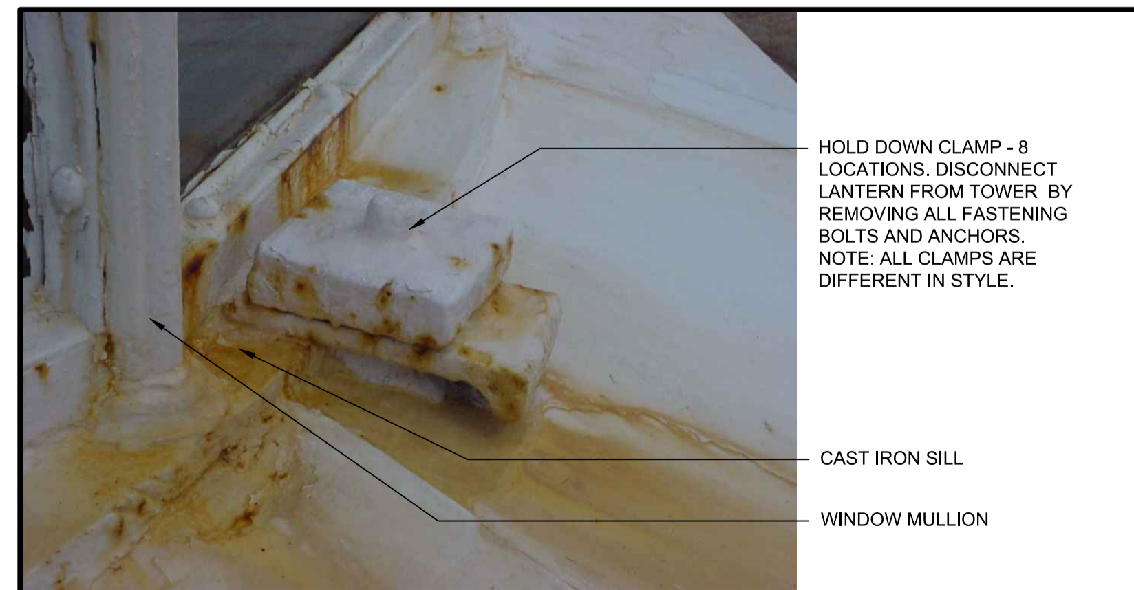
HOLD DOWN CLAMP AT DOME - TYP.
