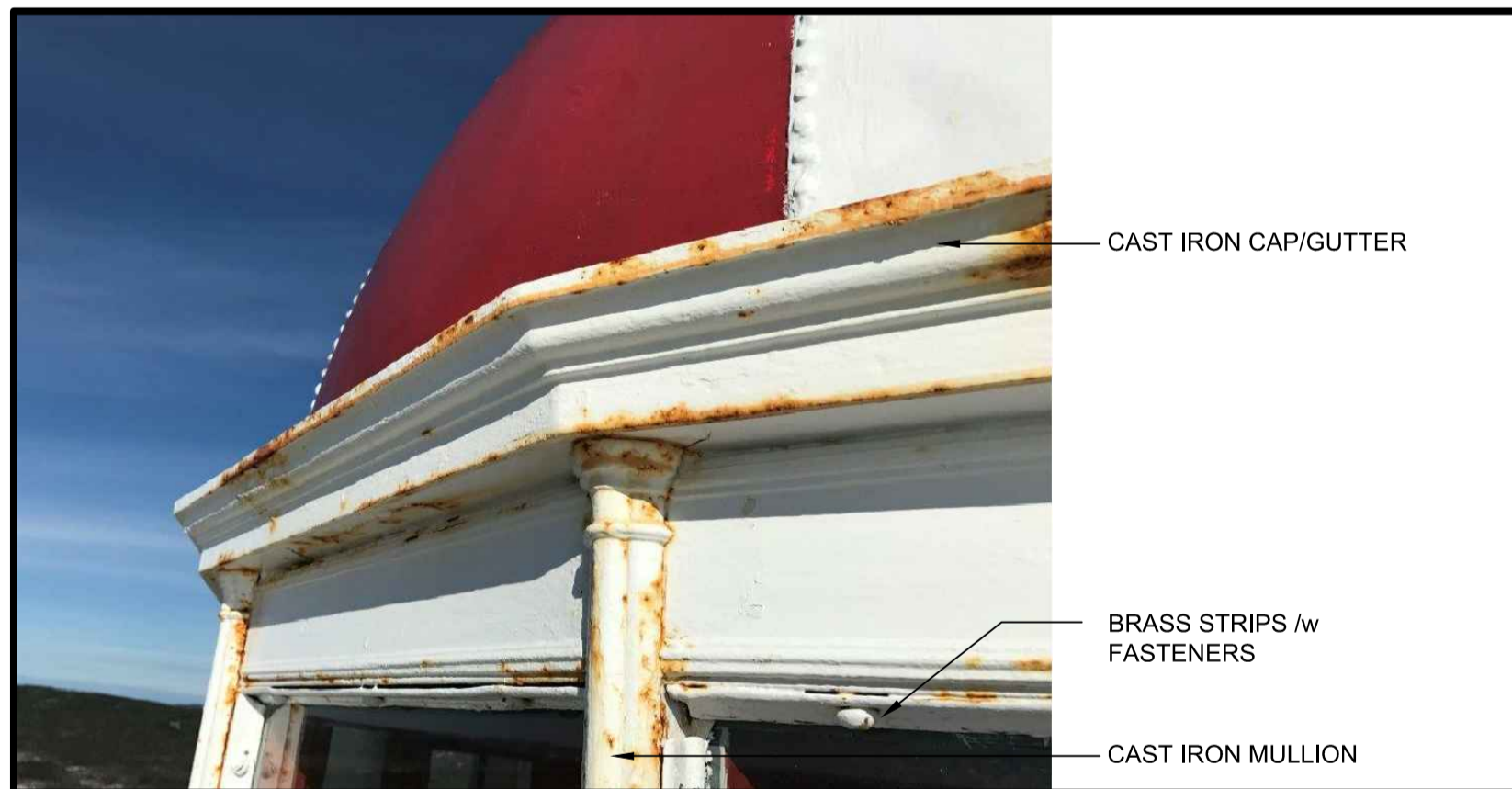
DOME - EXTERIOR GLAZING WINDOW HEAD
