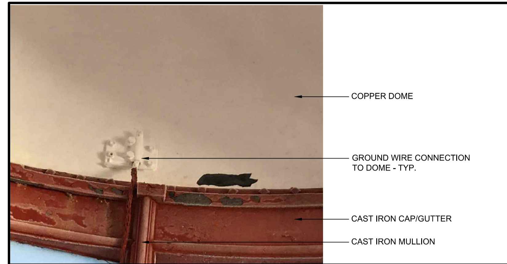
DOME - INTERIOR GLAZING HEAD AT GROUND WIRE
