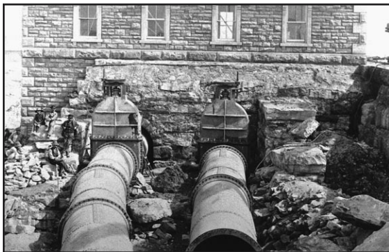
Penstocks supplying water to turbines in Powerhouse
