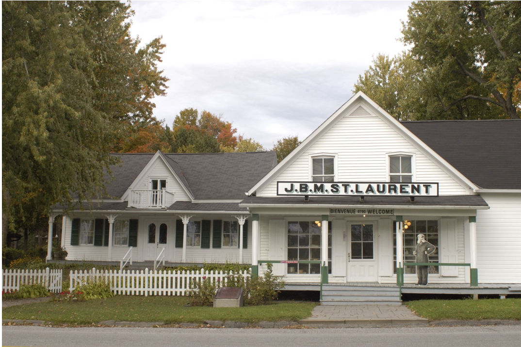
Louis S. St-Laurent National Historic Site
