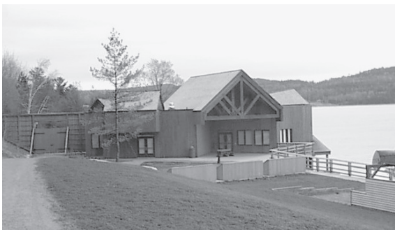
Reception and interpretation centre, exterior Public Works and Governmental Services Canada / C. Simard
