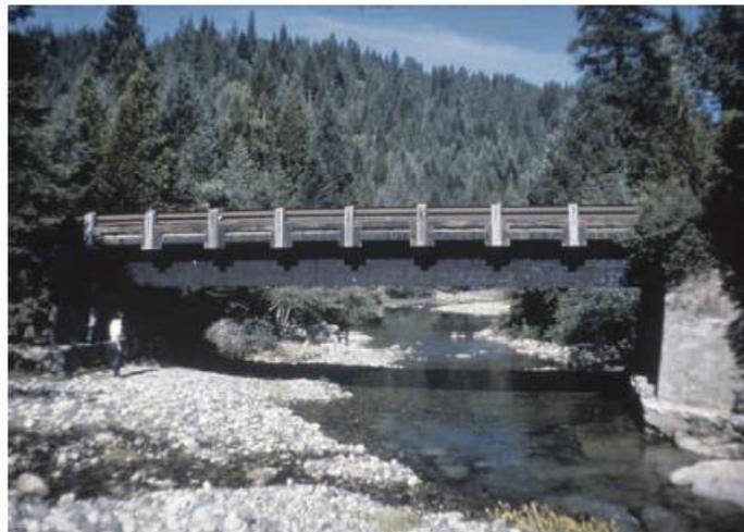
Figure 4.2 Oilborne preservatives are often used for treatment of glulam beams, such as in this bridge (Lebow and Tippie, 2001).
