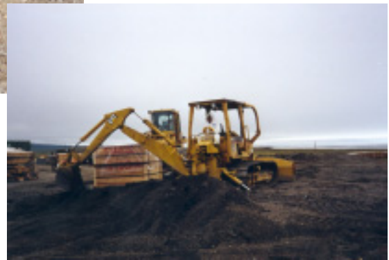
Removal of contaminated soil from Komakuk Beach.
