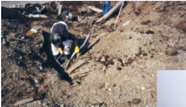
Cleaning up a landfill at Komakuk Beach.
