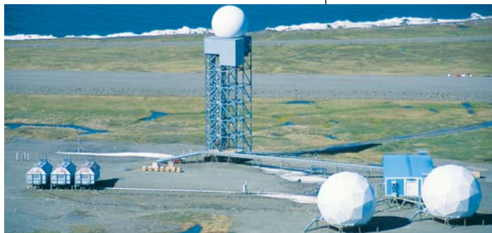
The site of the BAR-1 Distant Early Warning (DEW) Line station at Komakuk Beach after the clean-up in 1999 and 2000. PHOTO: IAN MCDONALD/PARKS CANADA.
