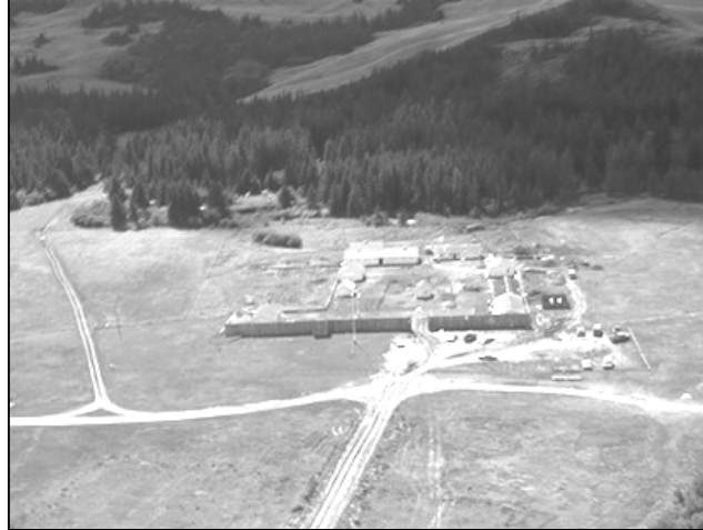
Figure 6. RCMP Remount Ranch, 1975. (Parks Canada)
