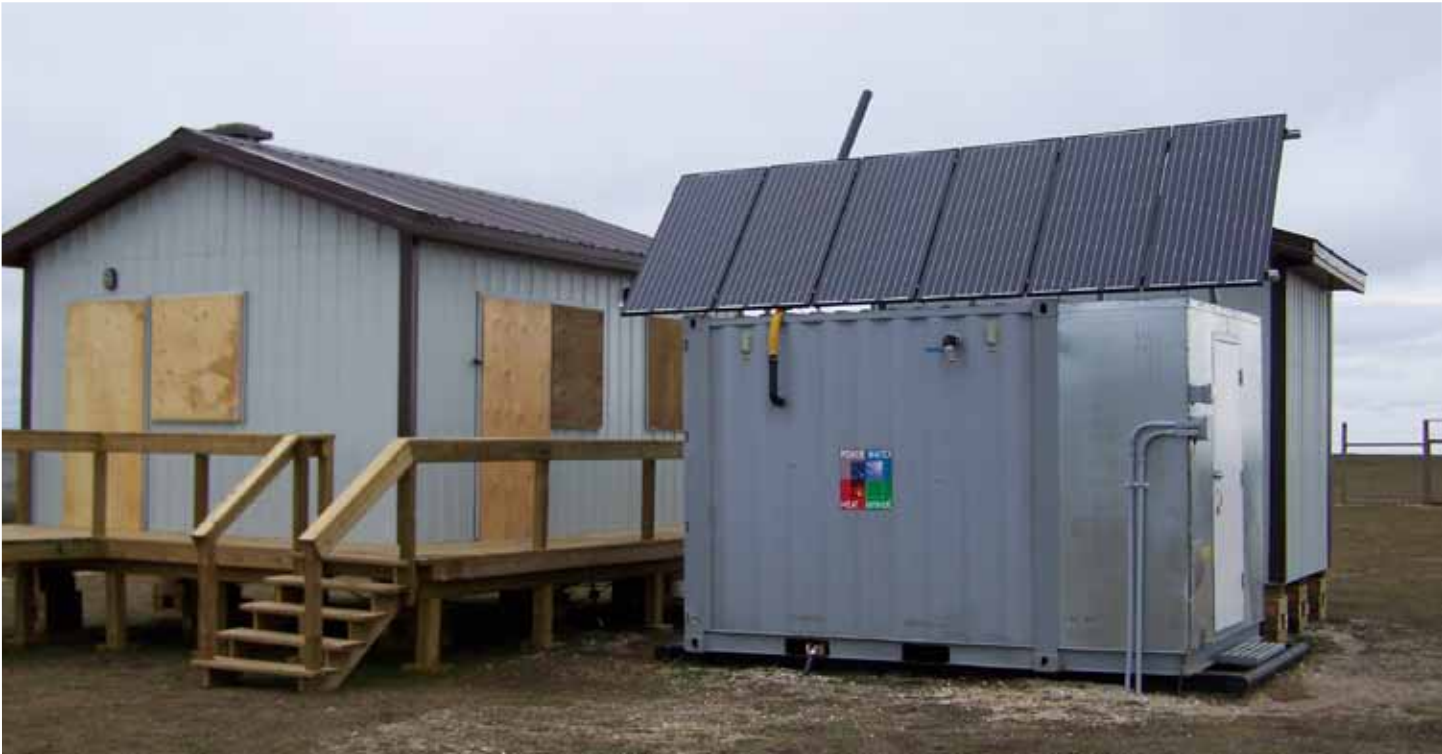
Figure 31: Water/wastewater treatment unit powered by solar source at Broad River in Wapusk National Park.
