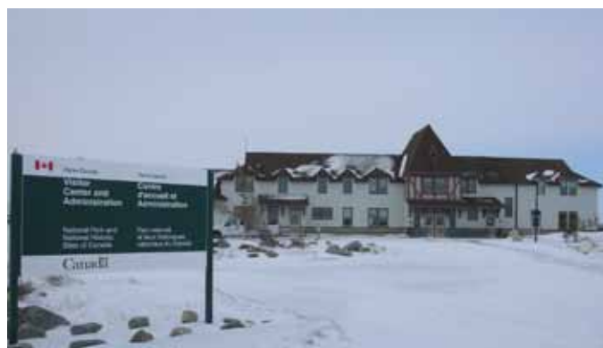
Figure 26: Parks Canada Visitor Centre and Administrative Office in Churchill.
