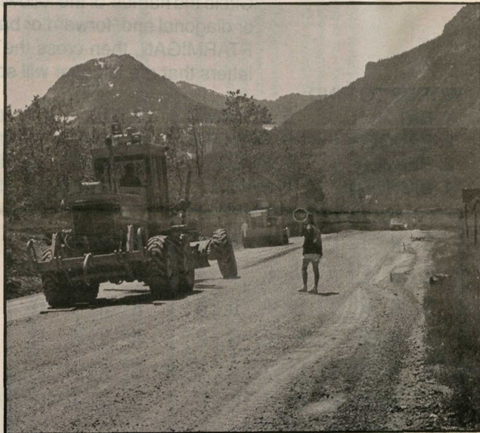
Road work in progress.
