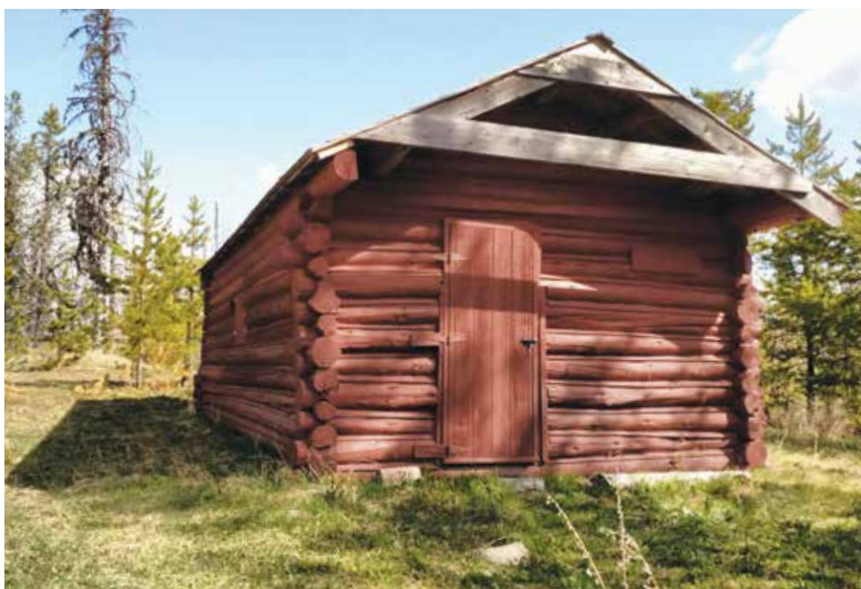
Historic preservation of the Matejka cabin completed by the Associates.
