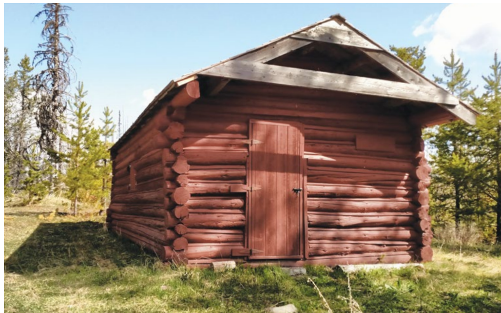
Historic preservation of the Matejka cabin completed by the Associates.
