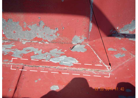
EXISTING FLASHING DETAIL FROM CUPOLA TO FLAT ROOF N.T.S.
