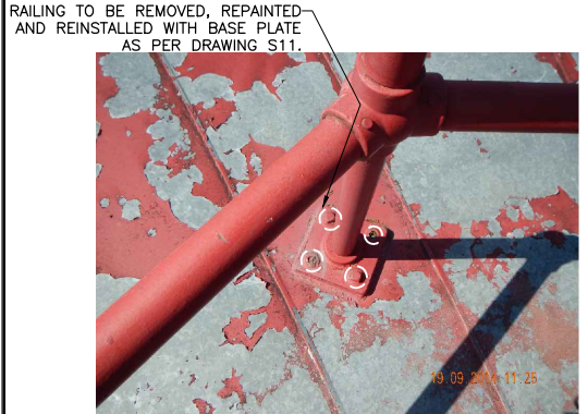
EXISTING RAILING CONNECTION TO ROOFING DETAIL N.T.S.
