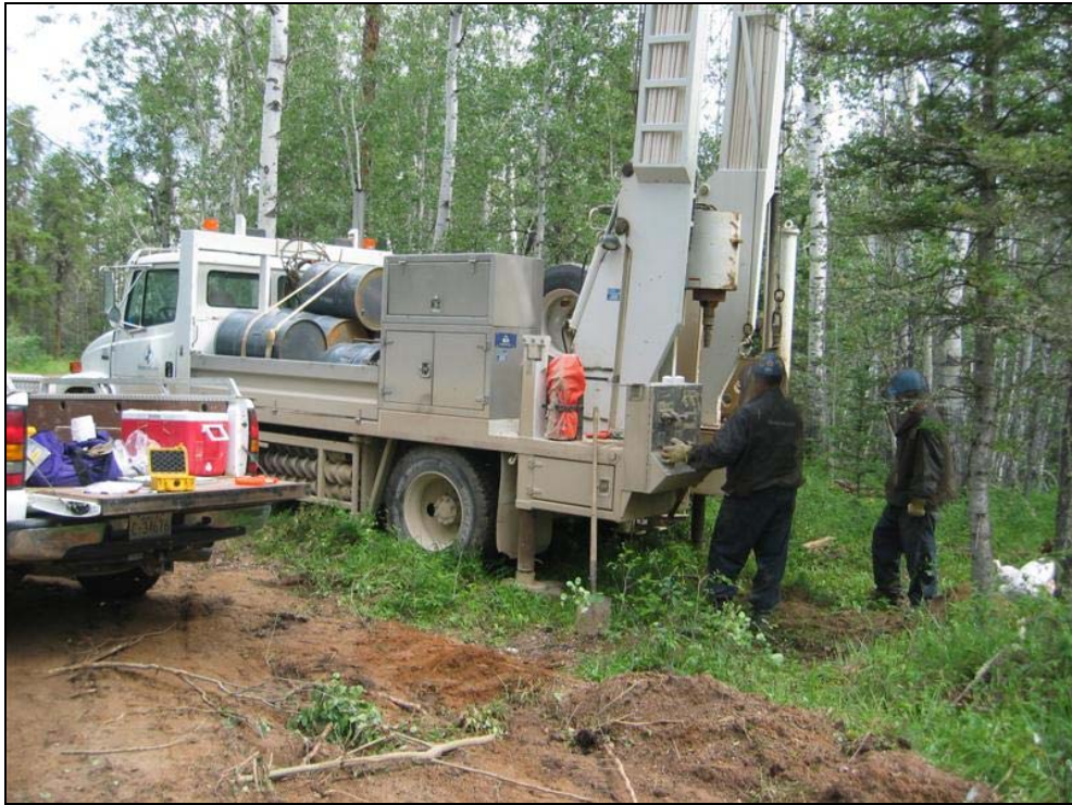
Photo 5: Drilling Monitor Well PL-MW2
