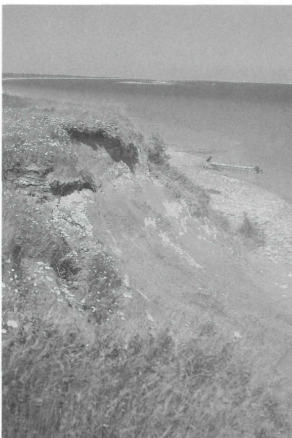
Riverbank erosion at the site.
