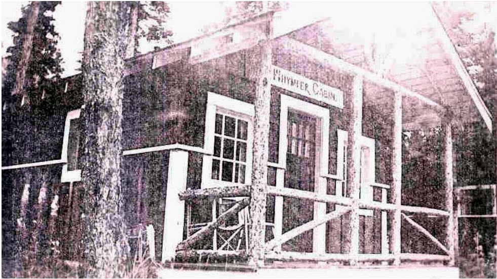
Figure 34. Although of poor quality, this September 1958 photograph shows the elaborate log verandah detailing that was reproduced with 2" x 4" lumber salvaged from dismantled Marble Canyon auto bungalows. The reproduced detailing is faithful to the original, with the exception that the steps are now located on the front rather than on the side of the verandah. ( LAC RG 84, A-2-a. Parks Canada, v. 1639, file K16-112-6, pt. 3. )
