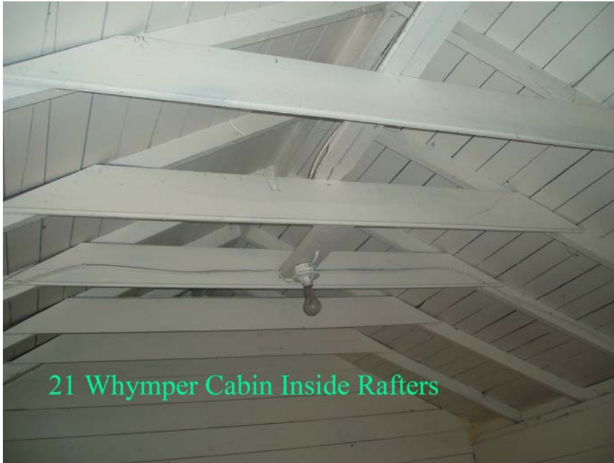
Figure 38. Whympers Cabin, interior, detail of rafters. ( Dennis Herman, Banff National Park, 2005. )
