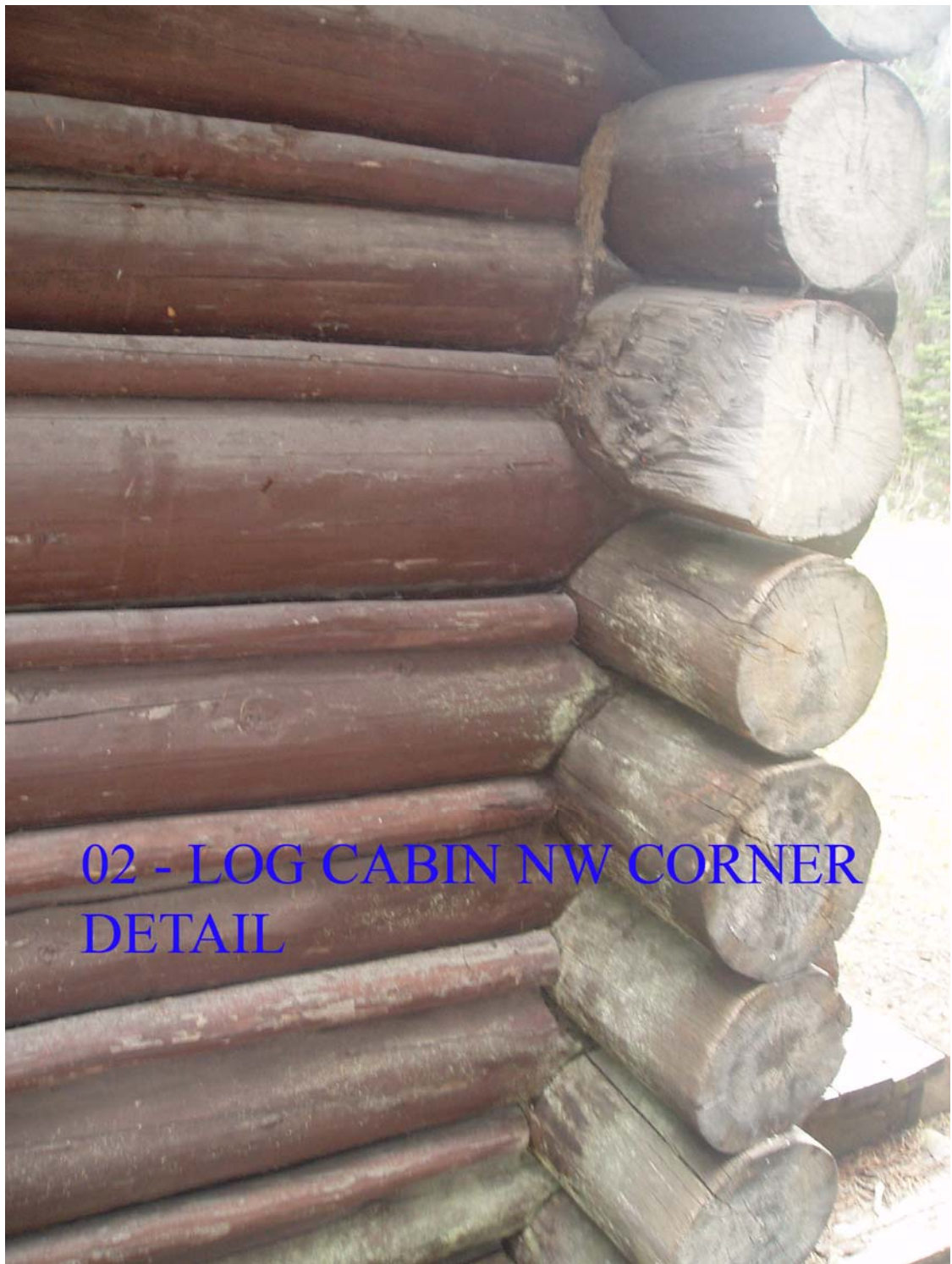
Figure 19. Old Log Cabin, detail of northwest corner showing saddle-notch log construction and stick batten treatment. (Dennis Herman, Banff National Park, 2005.)
