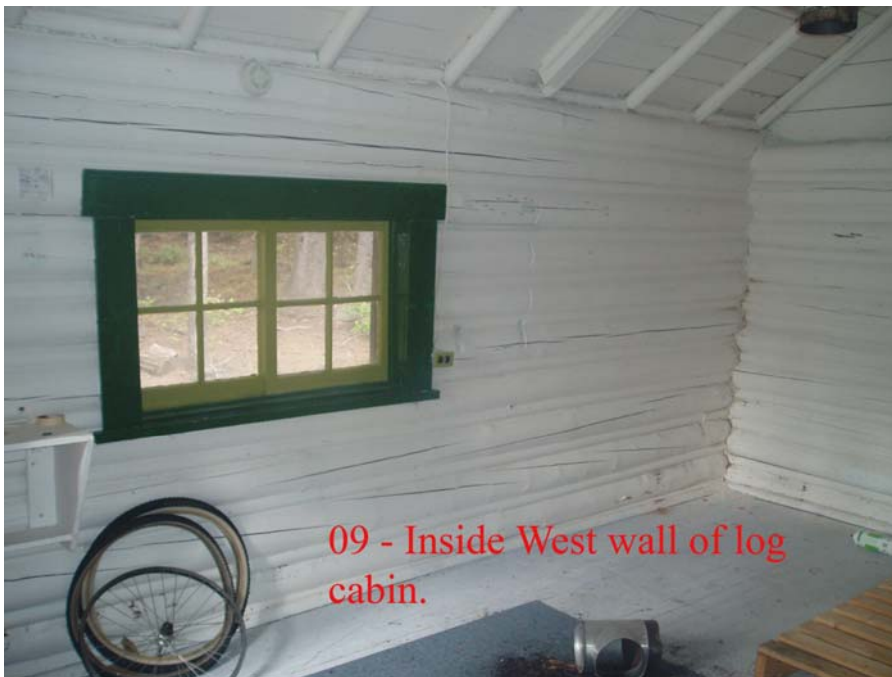
Figure 24. Old Log Cabin, inside west wall. ( Dennis Herman, Banff National Park, 2005. )
