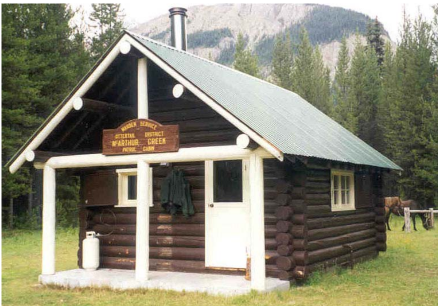
Figure 29. The McArthur Creek Patrol Cabin, Yoho National Park, built in 1957, is a late-arriving but typical example of a standard warden cabin in the mountain national parks. ( Cornell Wynnobel, "Application to the Federal Heritage Building Review Office: McArthur Creek Warden Patrol Cabin [and] Helmet Creek Warden Patrol Cabin," Federal Heritage Buildings Review Office, 1997: n.p. )
