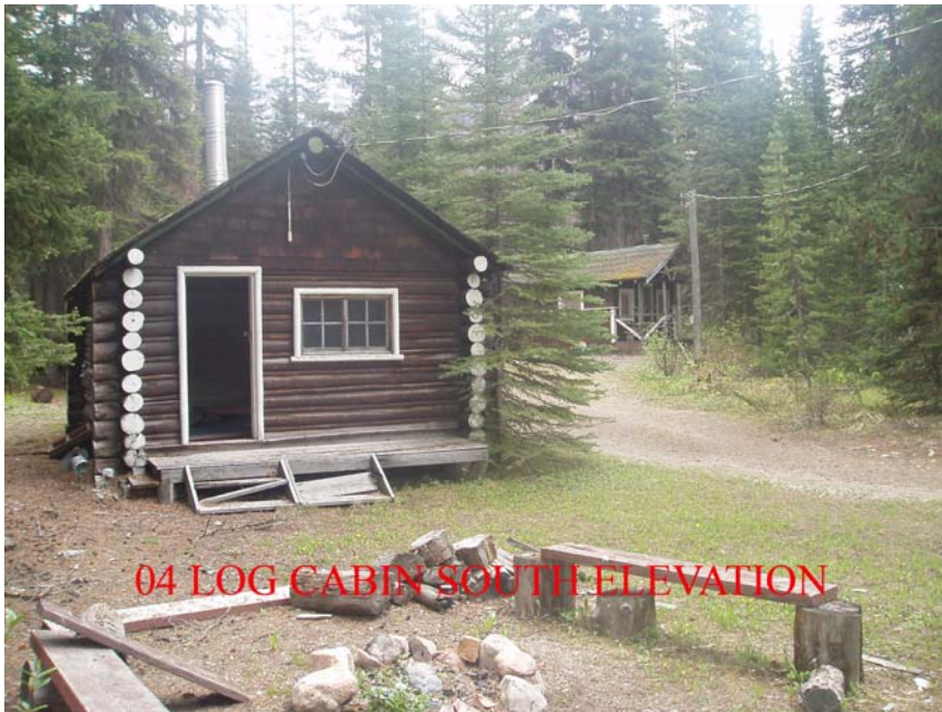
Figure 17. Old Log Cabin, south elevation. ( Dennis Herman, Banff National Park, 2005. )
