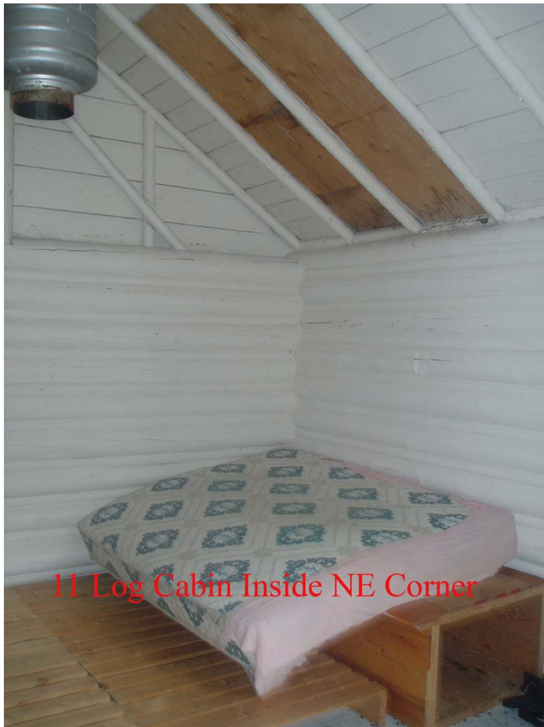
Figure 27. Old Log Cabin, inside northeast corner. Plywood patchwork appears to have been introduced to counteract a leaky roof. ( Dennis Herman, Banff National Park, 2005. )
