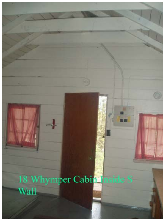
Figure 35. Whympier Cabin, interior, south wall. ( Dennis Herman, Banff National Park, 2005. )
