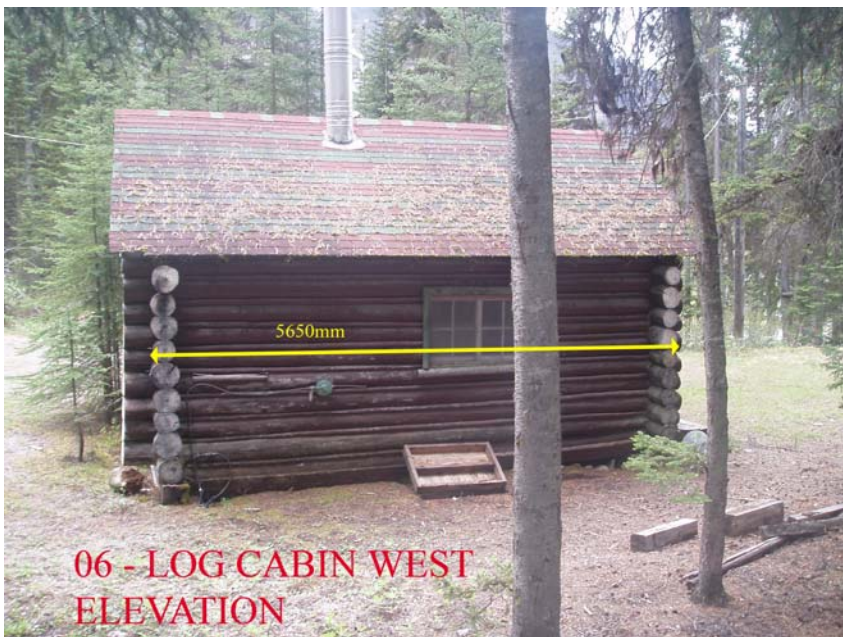
Figure 21. Old Log Cabin, west elevation showing roof shingle treatment. ( Dennis Herman, Banff National Park, 2005. )
