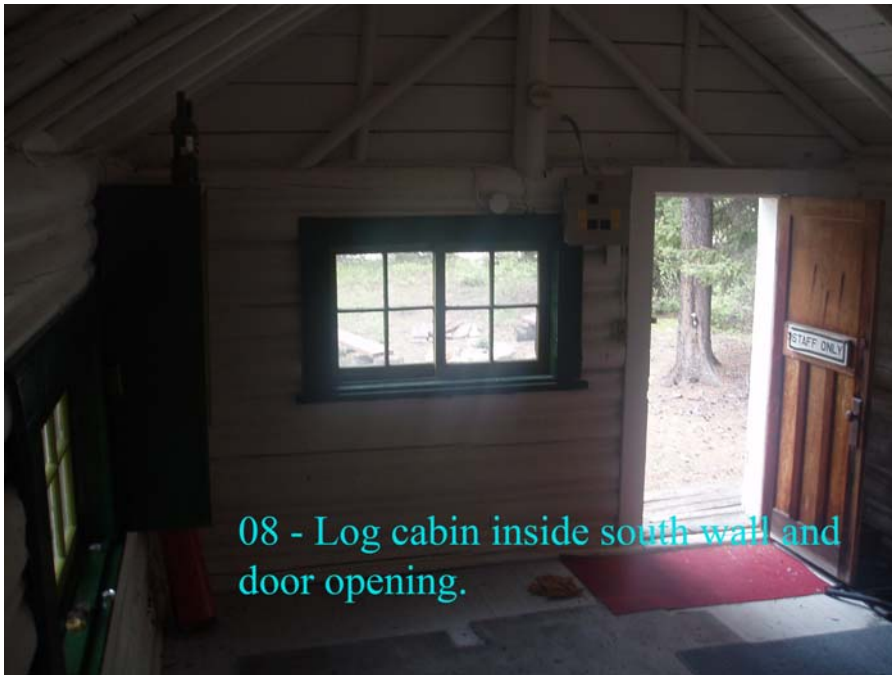
Figure 23. Old Log Cabin, inside south wall and door opening. ( Dennis Herman, Banff National Park, 2005. )
