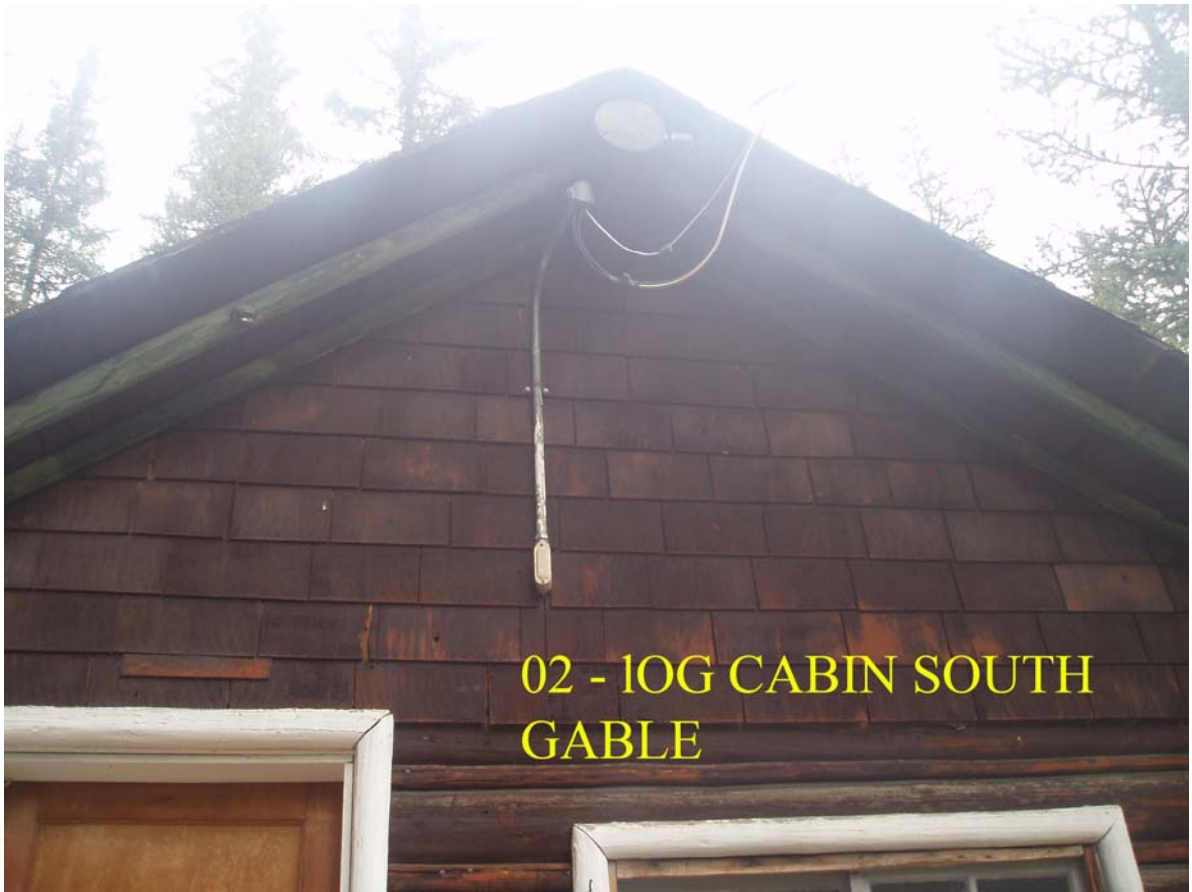
Figure 22. Old Log Cabin, detail of south gable showing cedar shingle treatment. ( Dennis Herman, Banff National Park, 2005. )
