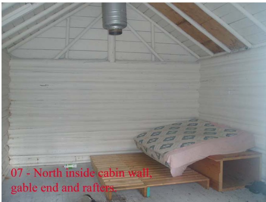
Figure 26. Old Log Cabin, north inside cabin wall, gable end and rafters. (Dennis Herman, Banff National Park, 2005.)
