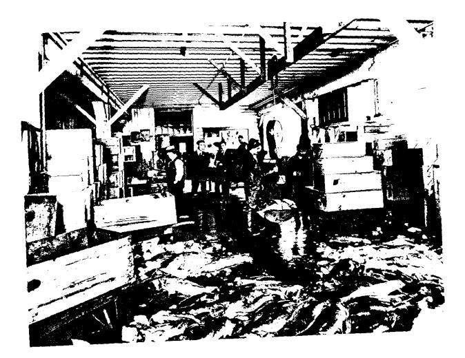
Photo 31 Ice making plant. Note cans being filled in foreground and tipper in background. Home Plant, 1918 (Canadian Fishing Co.)
