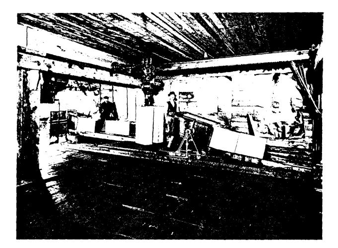
Photo 39 Ice Plant. Tipper discharging block of ice into freezer. Home Plant, 1985. (author)
