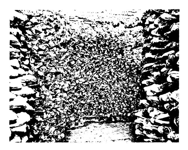
Photo 24 Fish in storage freezer. Note direct expansion pipe on ceiling. Home Plant, 1918 (Canadian Fishing Co.)
