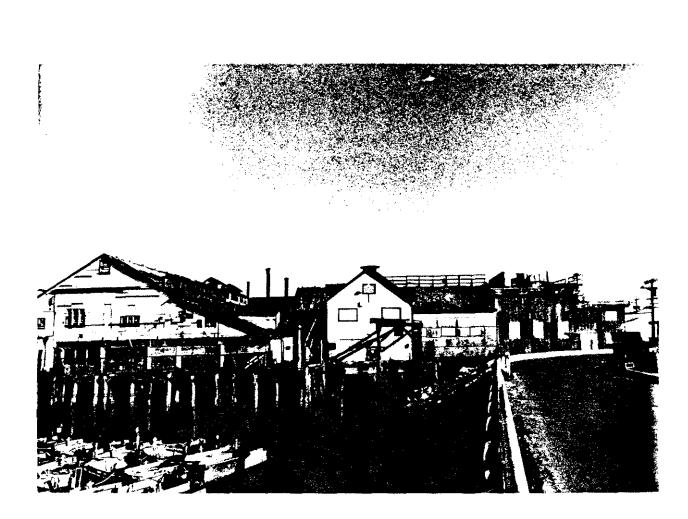
Photo 46 West side and front face of Gulf of Georgia ice house. Note timber framework on front face, which held ice chute to load ice directly into vessels, 1985. (author)
