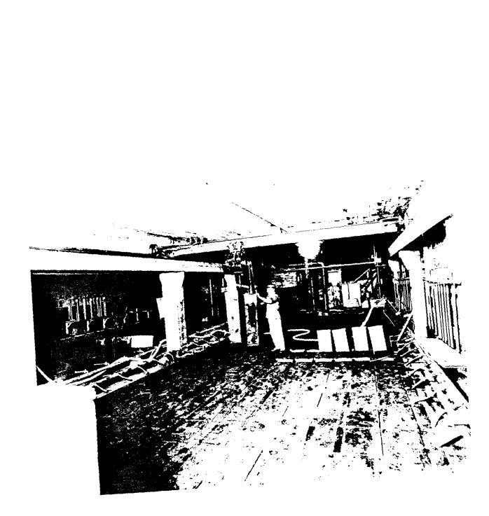
Photo 35 Ice making plant. Removing fresh ice from brine tank. Home Plant, 1985. (author)
