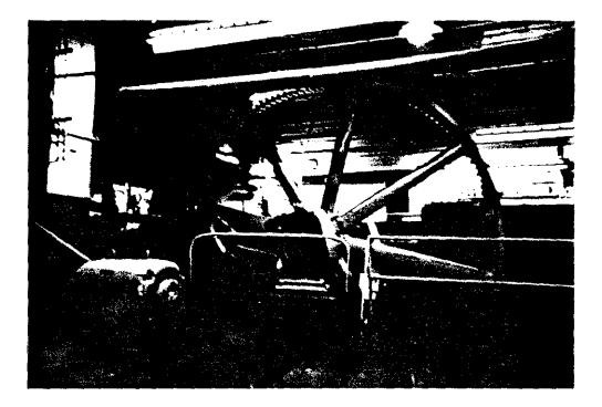
Photo 8 Rope drive and pulleys with generator in background, 1984 (author)
