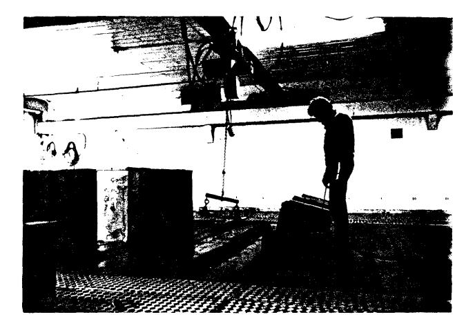
Photo 34 Ice making plant. Removing fresh ice from brine tank. Home Plant, 1918 (Canadian Fishing Co.)
