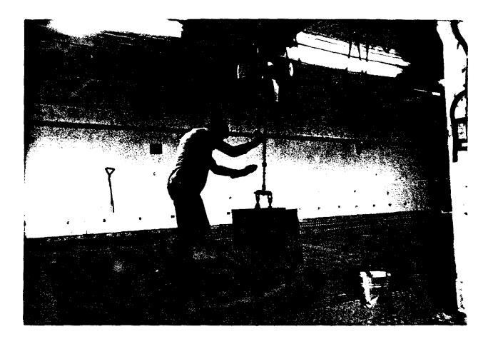
Photo 36 Ice plant. Moving ice to tipper. Note block of ice entering freezer, right side Home Plant, 1985 (author)
