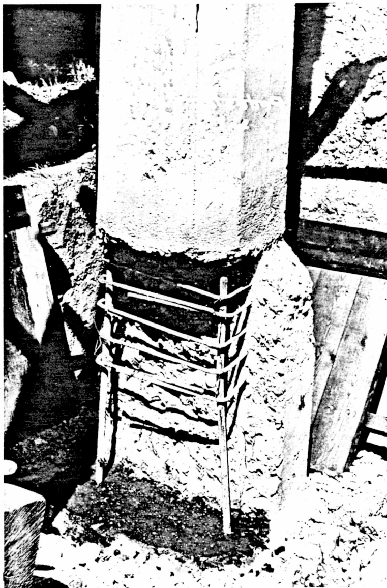
Illustration 19 Pedestal repair, 1927 (GAI NA-4389-36)
