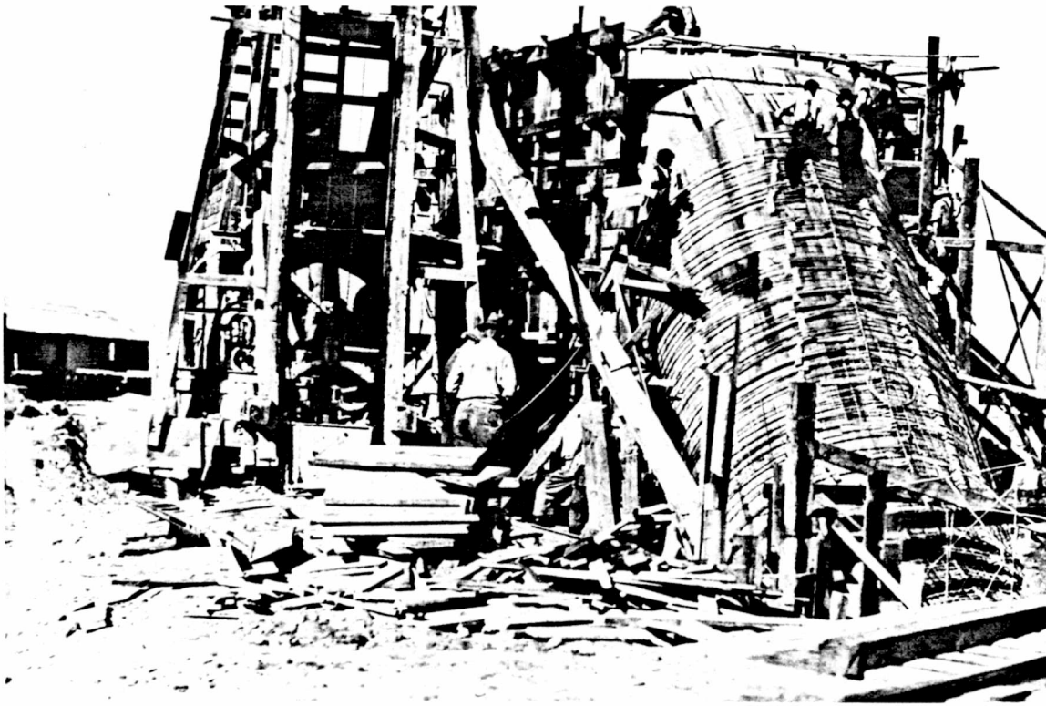
Illustration 7 Cement mixer at siphon, 1914 (GAI NA-2622-63)
