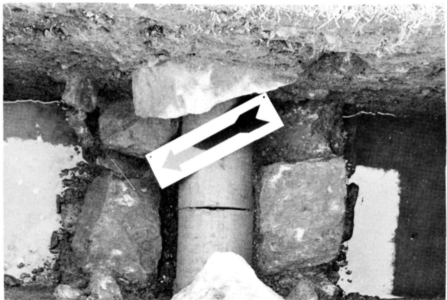
Appendix I - d. View of modern agricultural tile drain inside old British stone drain, with stones covering the drain protruding from both trench walls. 5G-63-M
