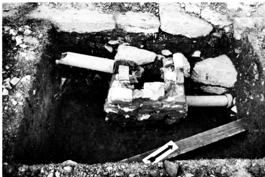
Appendix I - f. View of North east catch basin after excavation, showing two modern pipe inlets plus wood plank covering electric wiring. Surface runoff drain is seen at top of photograph. 5G-92-M
