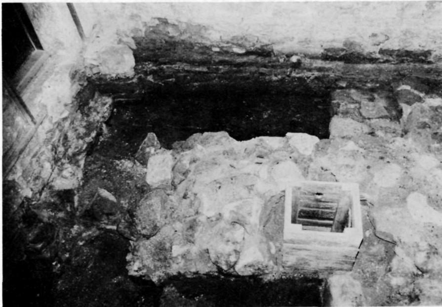
4. Section of foundations of original annex and structure predating original annex; inside present annex.
