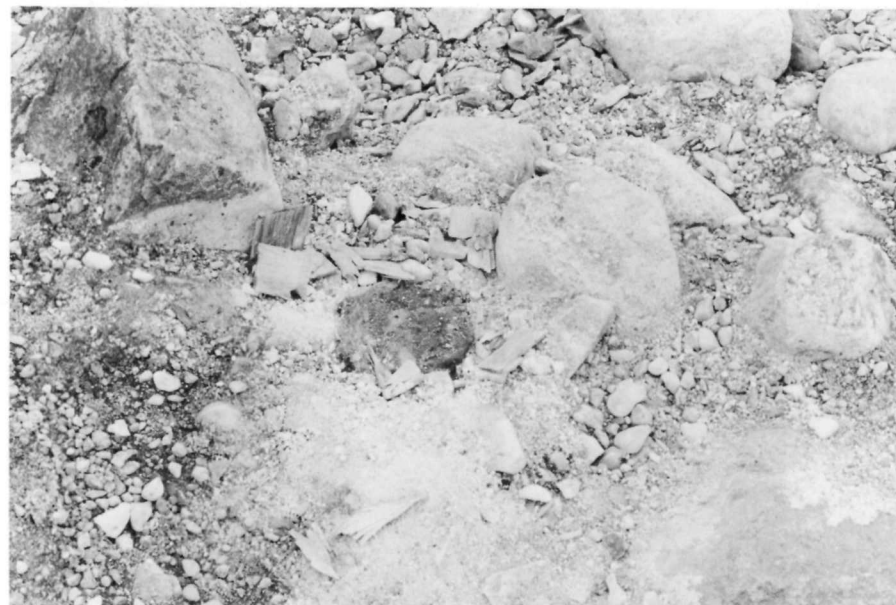
Figure 5. Corner post inside west parapet (refer to Figure 3b). (Photo 17K-43M).
