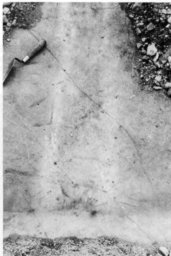
Figure 7. Mortar stains on bedrock, extending onto gravel (refer to Figure 3f). Facing south ( Photo 17K-28M ).
