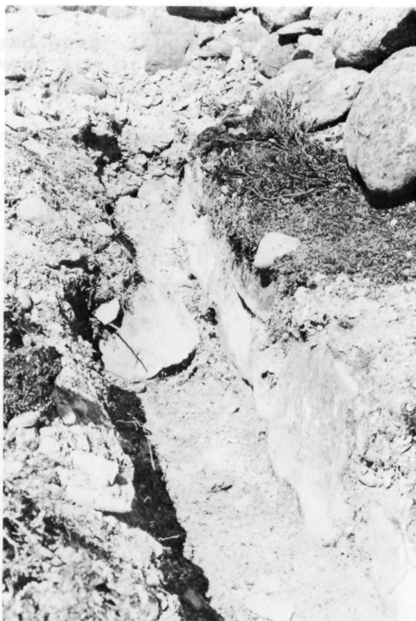
Figure 4. West parapet, exterior parapet line, showing mortared foundation stones. Facing north-northeast. (Photo 17K-33M)
