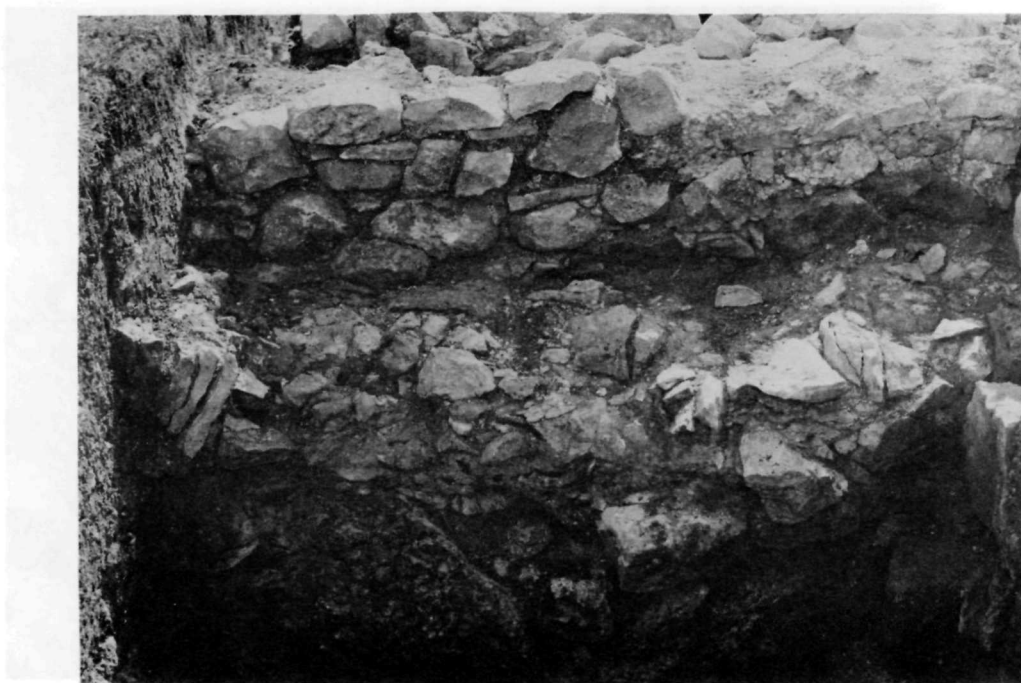
Figure 5. Construction details: south end of cellar's east wall, now extensively displaced, appears at bottom of photograph; east wall for renovation of original annex is directly above it. (Photo by author.)
