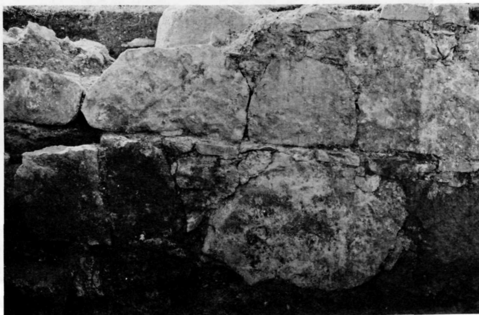
Figure 6. Construction detail: inner surface of south foundation in cellar area; note presence of a continuous line between courses, possibly representing a levelling course. (Photo by author.)
