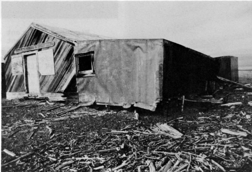
Figure 5. West wall of Northern Whaling and Trading Co. warehouse damaged by pack ice. (Photo by B. Ross.)
