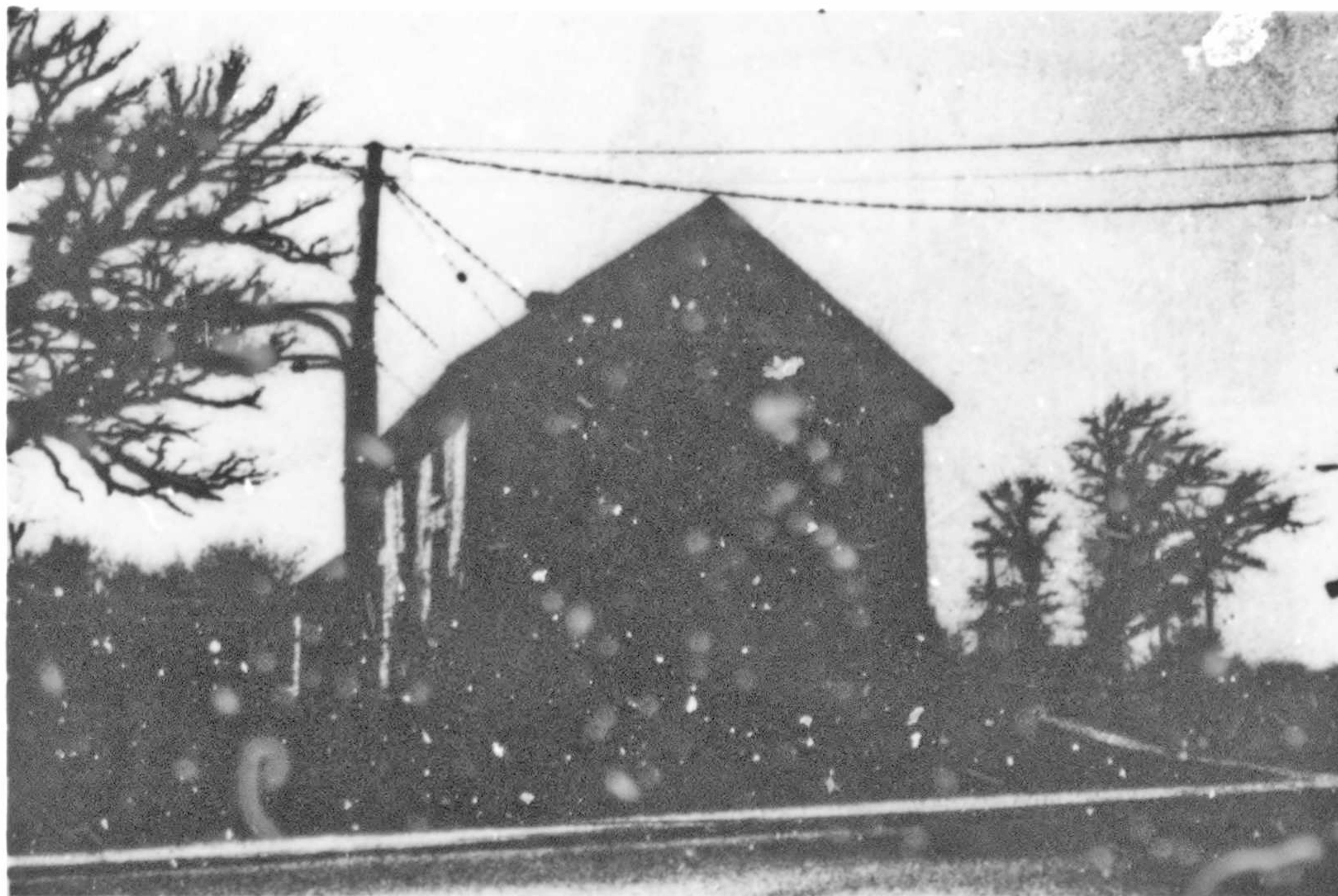
15 Former Depot School, Kingston, 1873. (CIHB, D. Johnson.)
