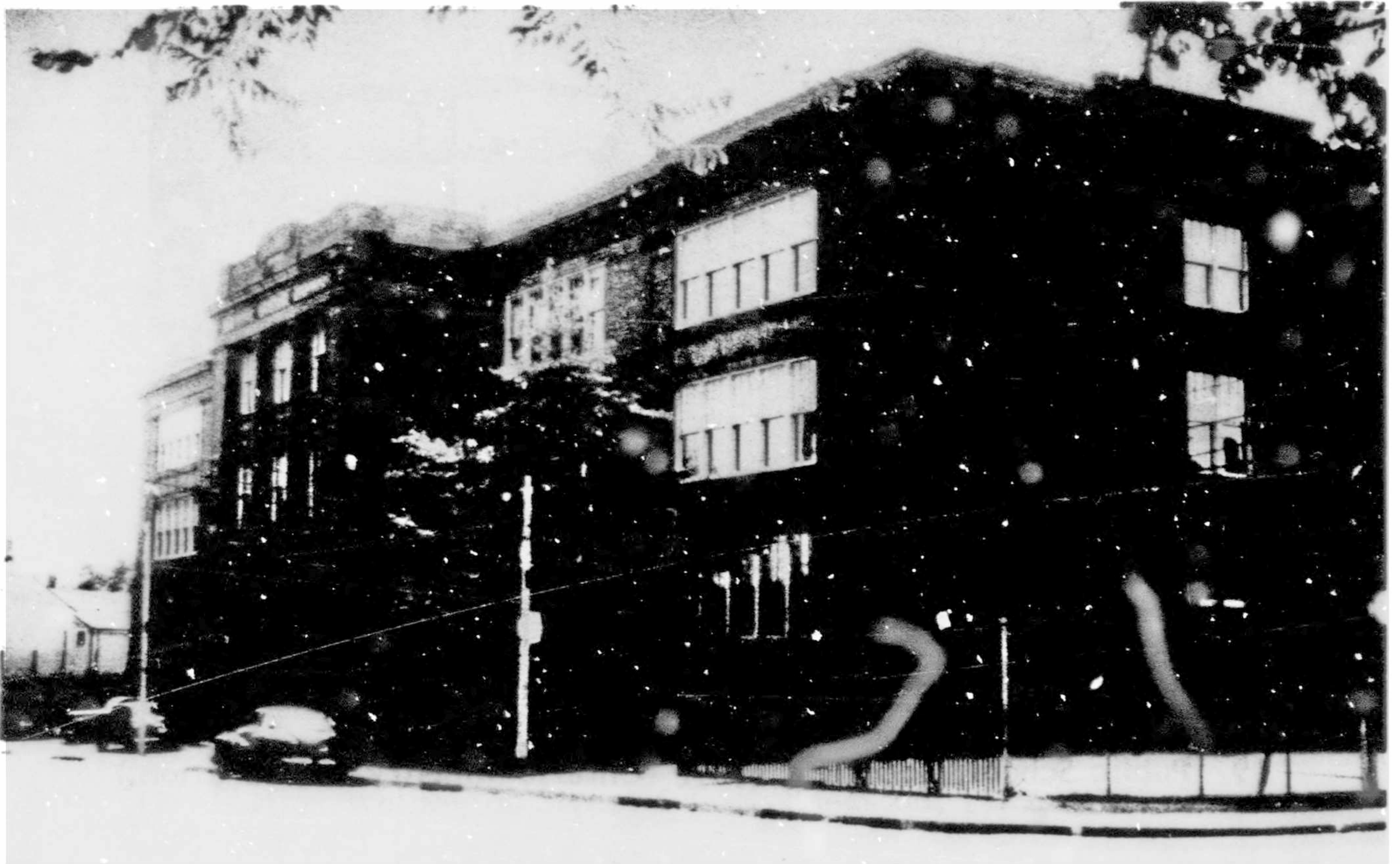
21 Givens Street Public School, Toronto, 1906. (Metropolitan Toronto Library Board.)
