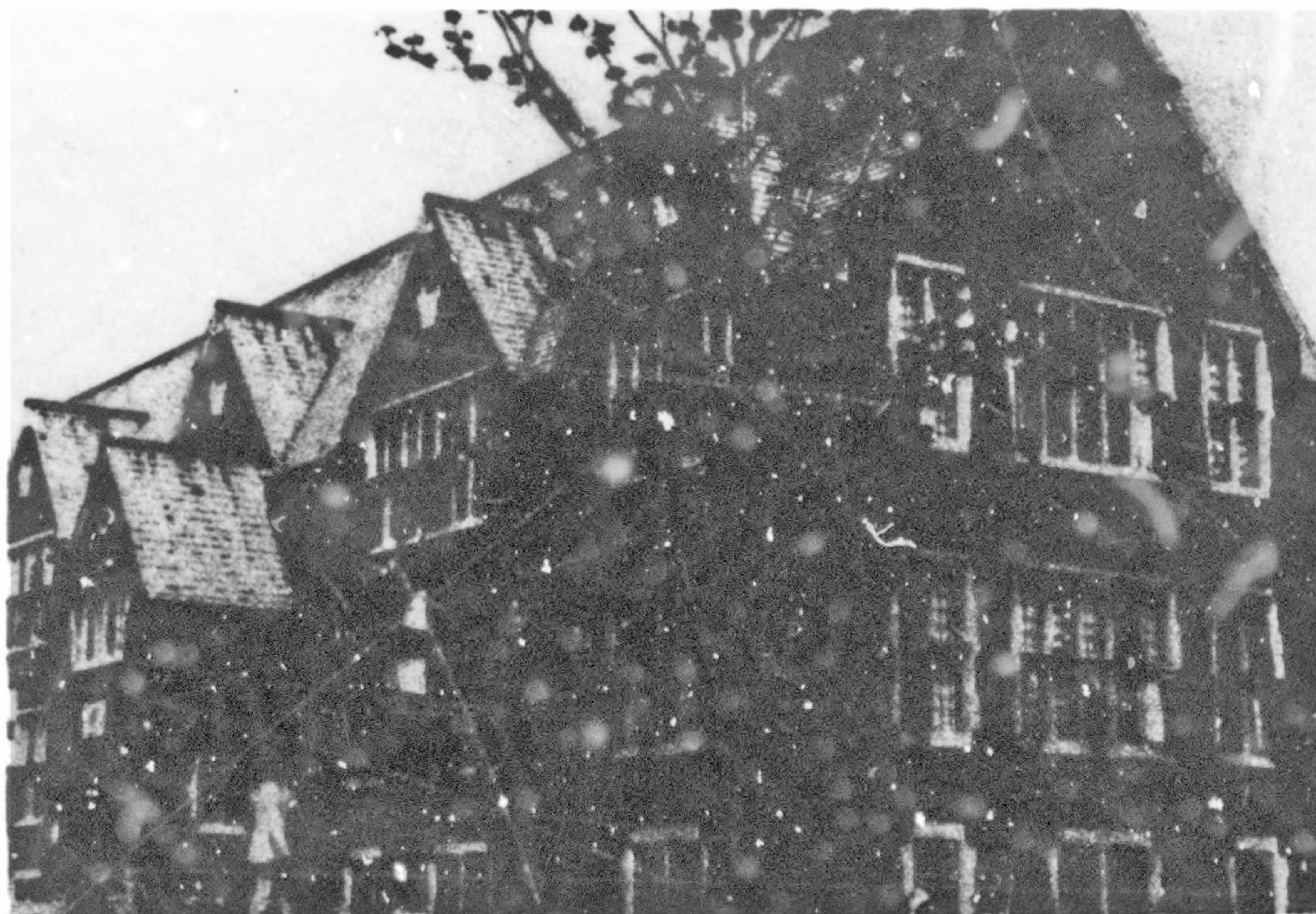
8 L'édifice Parkin, Upper Canada College, Toronto. (Mark Hord, Toronto.)
