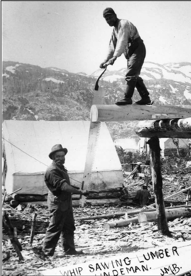
1898 April 25 - Must admit that a whipsaw is a man-killer. I know our saw does not run right. We only have 9 boards + have been sawing 3 days. We work like clockwork and do not seem to do anything. My back is most broken.
