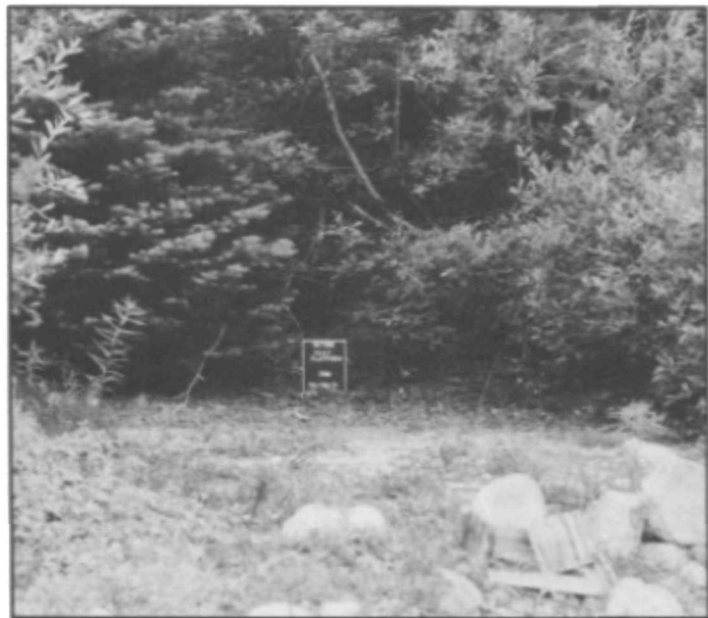
4 Tent platform recessed into hillside with dirt piled at front as an earthen and cobble retaining wall. Photo by P. Nieuwhof
