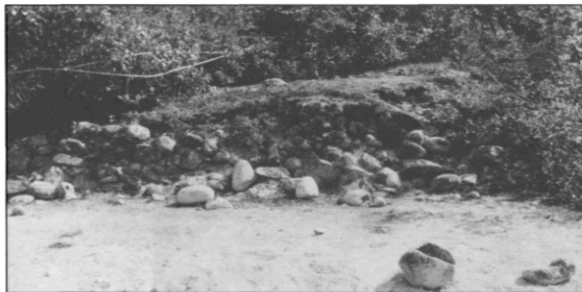
16 Loosened cobbles from a retaining wall due to visitors inadvertently walking over the historic wall. This action will eventually lead to the collapse of the wall and a loss of integrity of the landscape.
