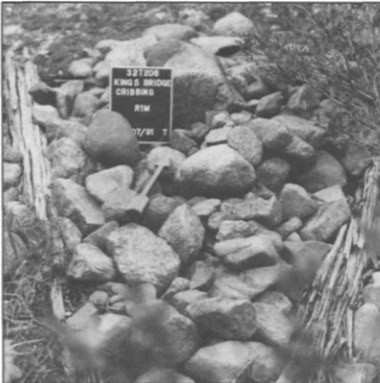
8 Detail of one of the 11 rock cribs of the King's Bridge over One Mile Creek. Photo by P. Nieuwhof
