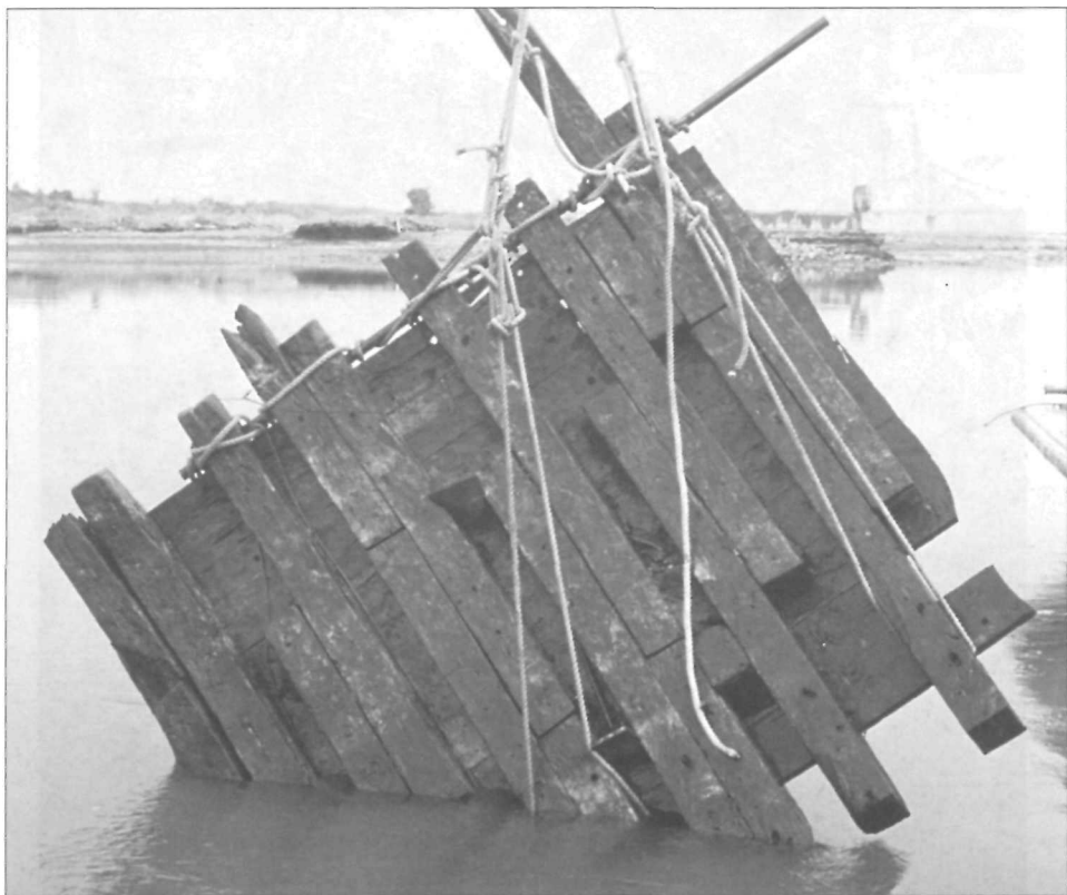
12 Starboard section of the hull of the Machault . Department of Canadian Heritage.
