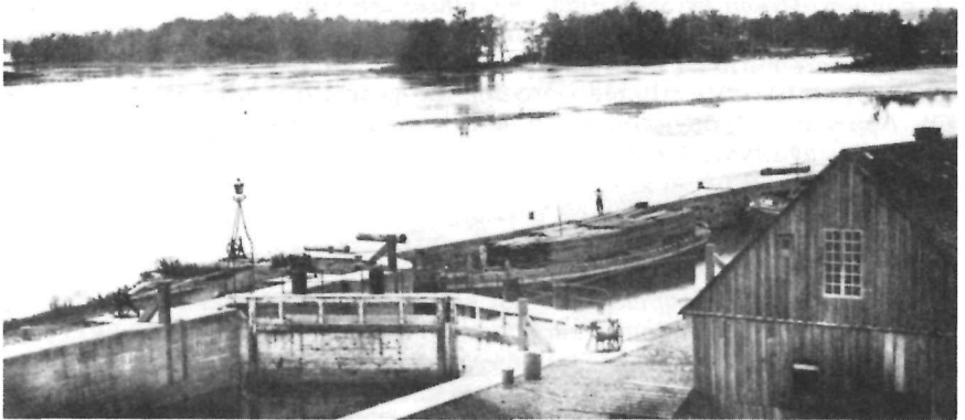
18 Barge loaded with lumber preparing to leave Ottawa River canal system at St. Anne's lock. One of these barges could carry up to 300 000 feet of lumber. (Undated, Public Archives of Canada.)
