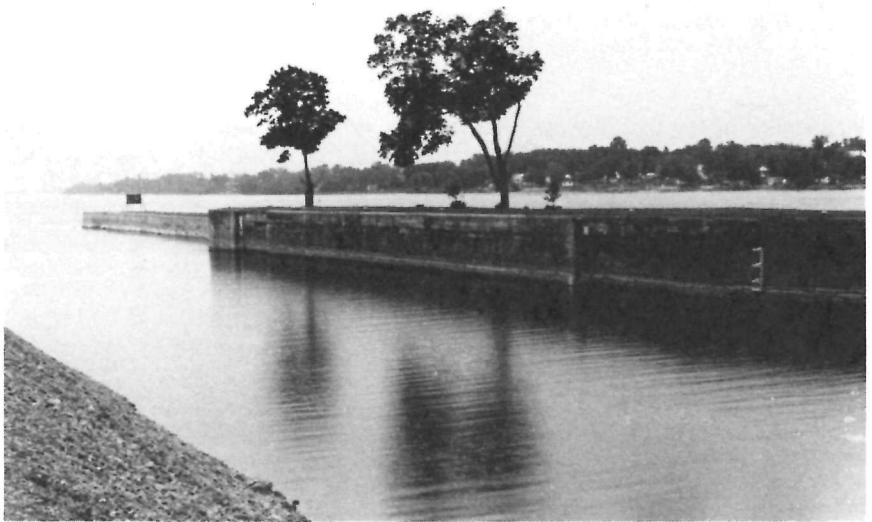
15 The south chamber wall (lateral wall) of lock No. 1 of the second Carillon Canal was saved from demolition when the present Carillon lock was built. It now forms part of the end of the downstream wharf leading to the present Carillon lock.
