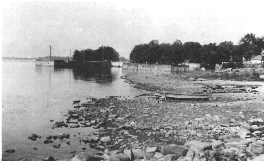
13 Downstream entrances to first two Carillon canals in 1914. At left, entrance to second canal, in operation from 1882 to 1960. At right, entrance to old military canal of 1834, remnants of which can still be seen.
