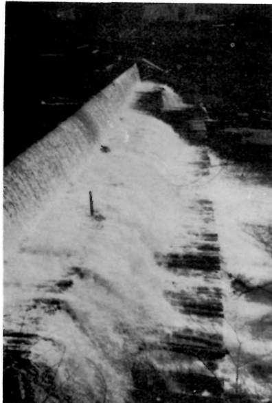
Dam on Upper Salmon River near Alma, looking east to show flow of water over entire face of dam. May 16, 1948.
