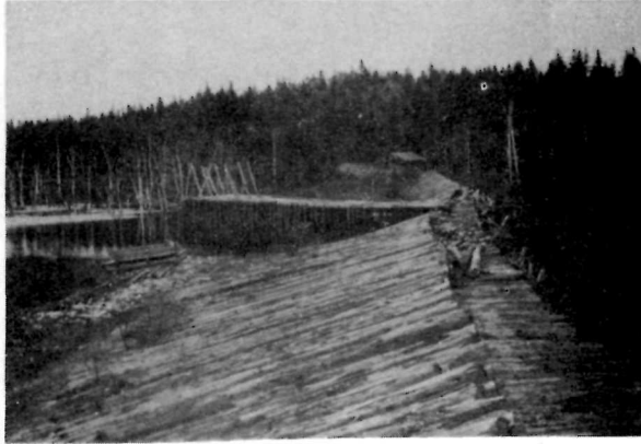
"Driving" dam on Drummond stream as seen from west end looking east. Structure to left of dam face in centre of dam is control for quick release of water for log driving. May 24, 1948.
