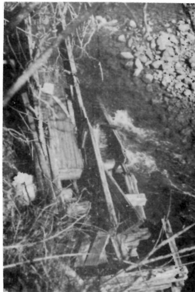
Unserviceable fishway at west end of dam on Upper Salmon River as seen from south end. May 16, 1948.
