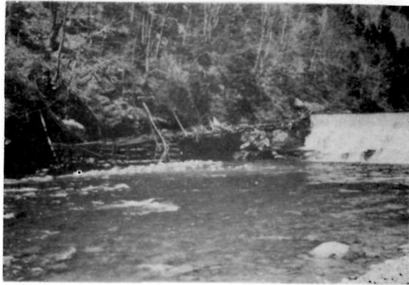
Unserviceable fishway at west end of dam on Upper Salmon River. May 16, 1948.
